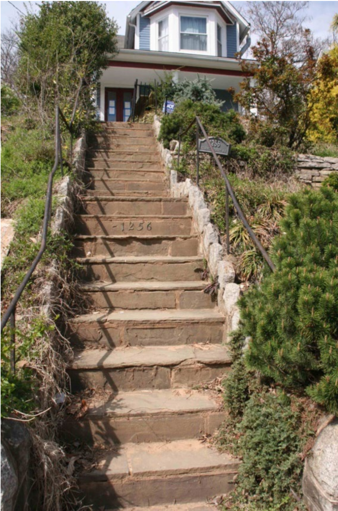
Photo 2 (DC_Slowe Burrill House_0002)
