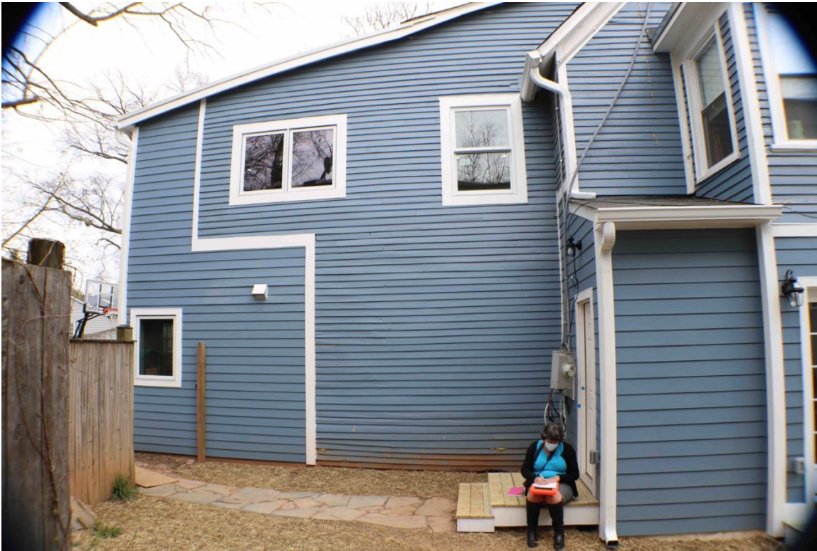
Photo 6 (DC_Slowe Burrill House_0006)
