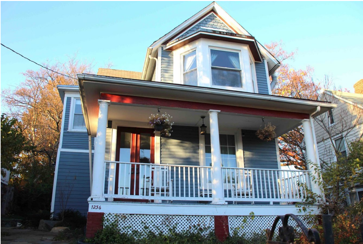
Photo 3 (DC_Slowe Burrill House_0003)
