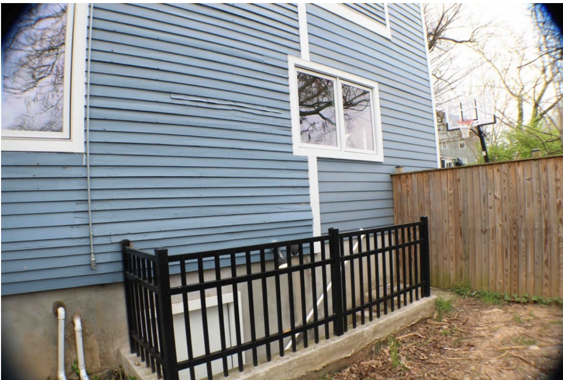
Photo 9 (DC_Slowe Burrill House_0009)
