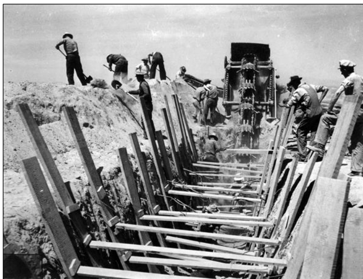
Workers of Japanese ancestry are using a ditch-digging machine to excavate for water pipes and sewer lines at Poston.
