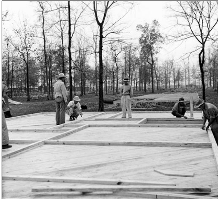
Apartments are being built for the administrative staff at Rohwer in this 1942 photo. The wood frame construction made it fairly easy to remove the buildings after the war, so the land could be returned to cultivation.
