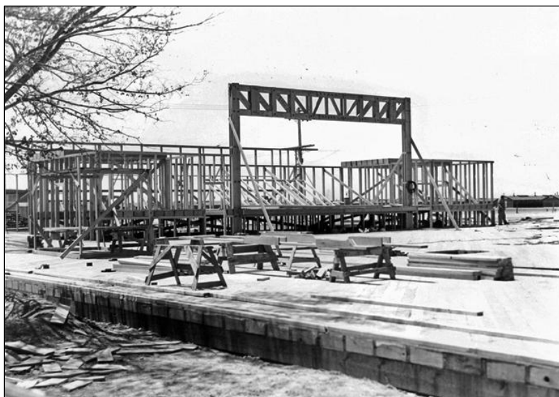
The first truss is installed for the high school at the Topaz Relocation Center. WRA photo by R. Bankson, July 1943 Courtesy of the U.S. National Archives and Records Administration
