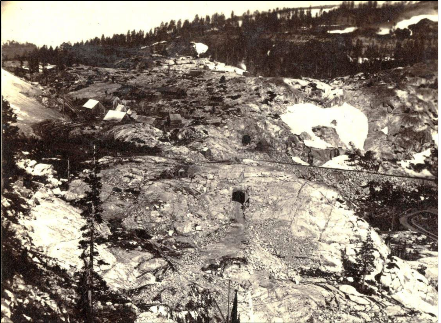
Figure 11. “East Portals of Tunnels No. 6 and 7 from Tunnel No. 8,” Photograph no. 202, A.A. Hart for Central Pacific Railroad Company, c. 1865-1868. Overview of Summit Camp area taken facing west from above Tunnel No. 8 showing the east portals of Tunnels No. 6 (back center) and No. 7 (center), China Wall (foreground), Dutch Flat Donner Lake Road, (upper right), and Summit Camp (upper left). Department of Special Collections and University Archives, Stanford University.
