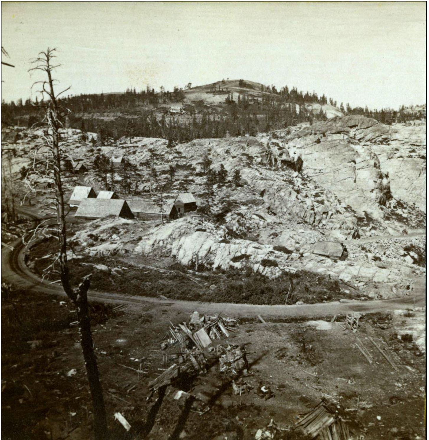
Figure 9. “Camp near Summit Tunnel – Mt. King in the Distance,” Photograph no. 116, A.A. Hart for Central Pacific Railroad Company, c. 1865-1869. View facing northwest with Dutch Flat Donner Lake Road in foreground and Summit Camp at the left. Department of Special Collections and University Archives, Stanford University.
