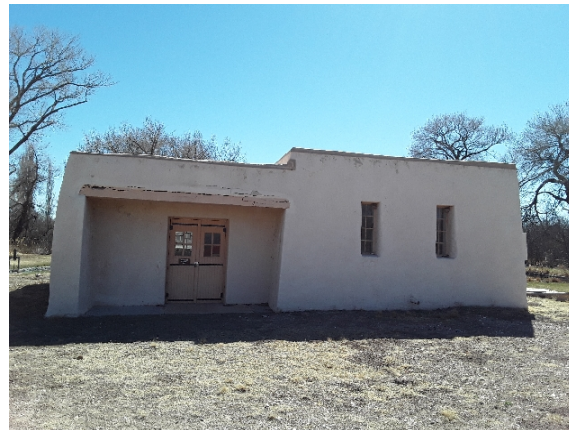
2020_CAVE_15602_RS Pump House_Front.jpg
