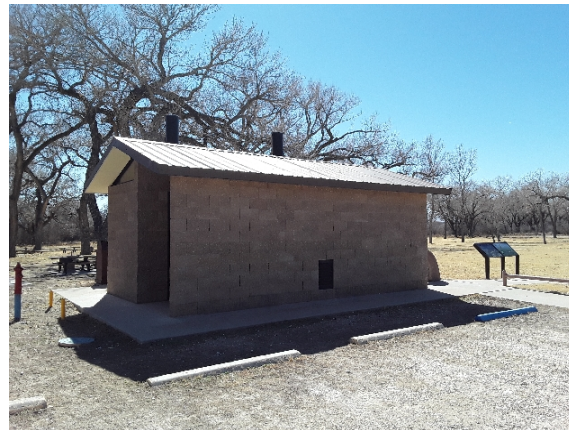
2020_CAVE_82424_RS Double Vault Toilet_Front.jpg
