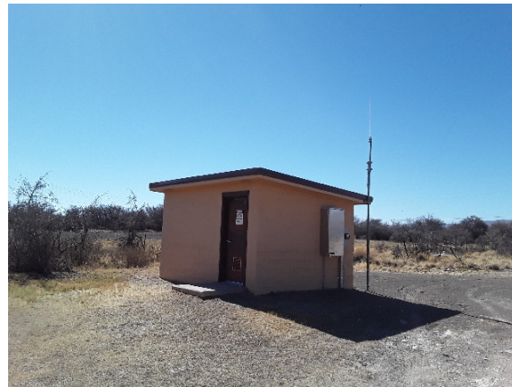
2020_CAVE_81658_RS Well House_Front.jpg
