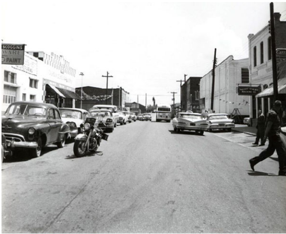
FIGURE 2-7. The Greyhound bus (center) on Gurnee Avenue about to turn right onto W. 10th Street on May 14, 1961. Birmingham Civil Rights Institute.
