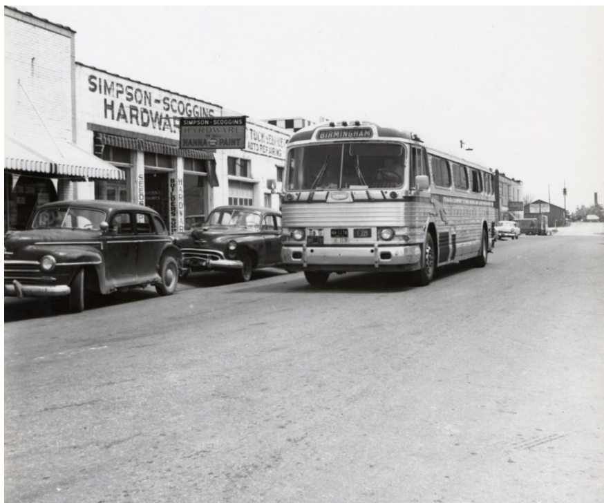
FIGURE 4-7. View looking south on Gurnee Avenue at the Greyhound bus as it approaches W. 11th Street, where it will turn right, then right again to enter the alley behind the bus depot. Courtesy of the Birmingham Civil Rights Institute.
