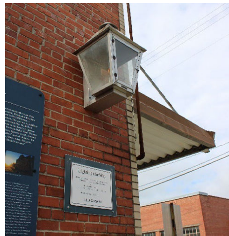
FIGURE 3-33. Stainless steel gas lantern mounted by Alagasco, 2021. Laura Knott.
