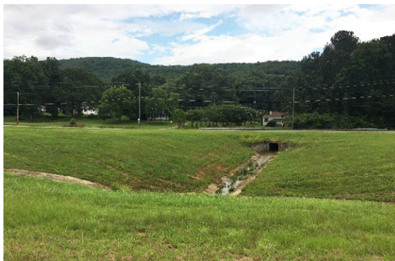
FIGURE 3-24. Looking north at a portion of the large stormwater drainage structure that crosses Parcel 54, 2021. Laura Knott.
