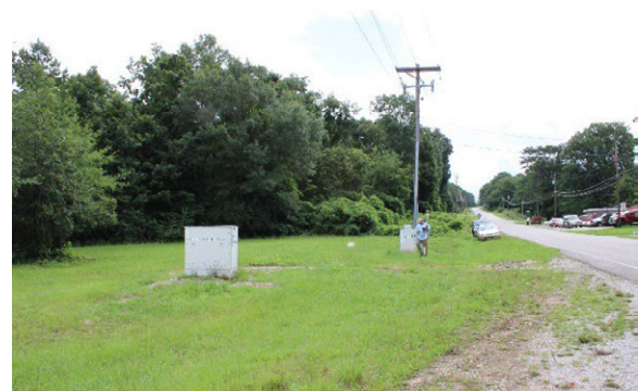
FIGURE 3-23. Utility box that serves the electrical lines that cross the Bus Burning Site, 2021. Laura Knott.
