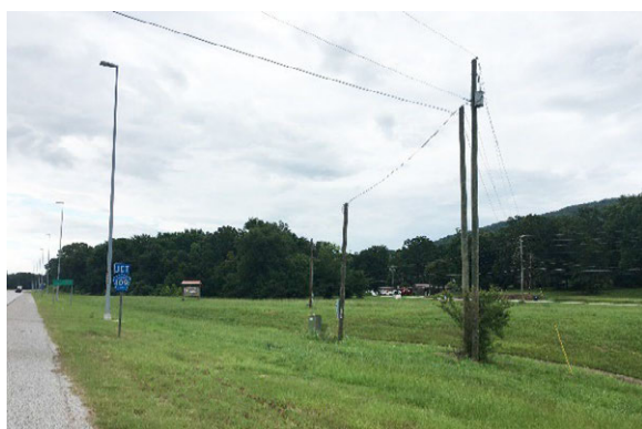
FIGURE 3-37. Utility poles, light standards, and information signs in Parcel 54 of the Bus Burning Site, looking east, 2021. Laura Knott.
