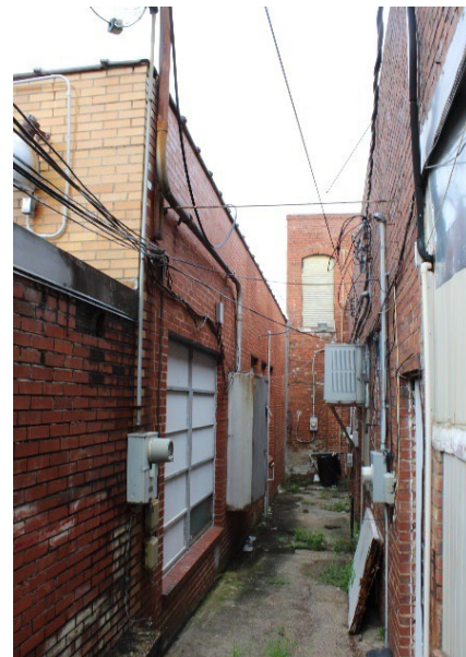
FIGURE 3-19. Looking west into the areaway with the Bus Depot building to the left, 2021. Laura Knott.
