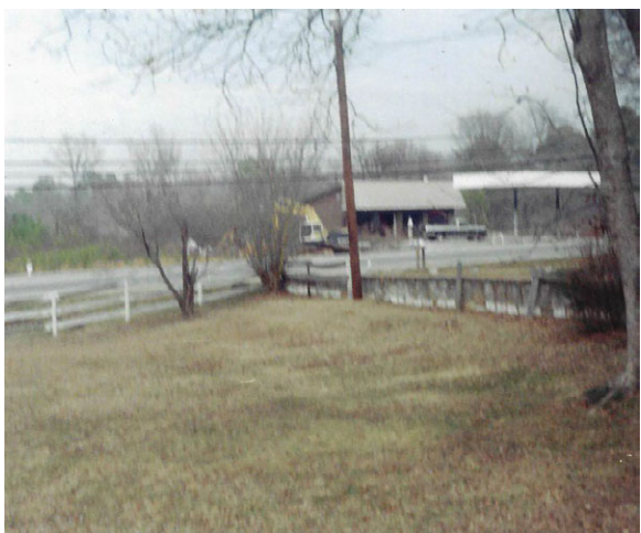
FIGURE 2-29. View of the remodeled grocery store ca. 1980s taken from a neighboring residence to the southwest. National Park Service.
