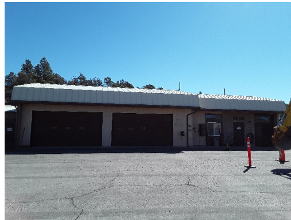
2021_GICL_90736_Maintenance and Storage_Front.jpg
