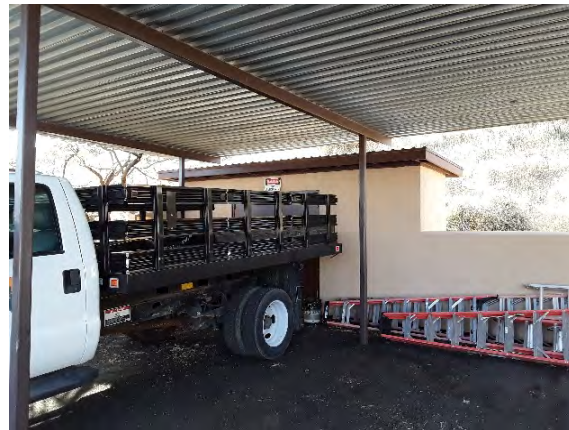
2021_TONT_75796_Powered Equipment Shed_Front.jpg
