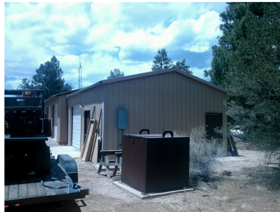
2018_ELMA_40672_Pump Hose Fire Cache_Front.jpg
