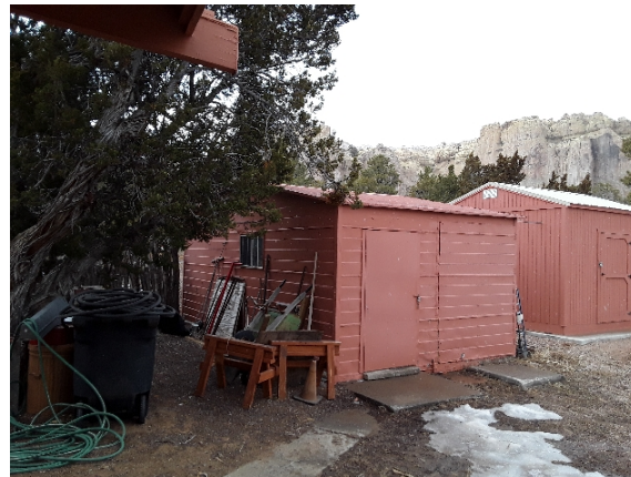
2021_ELMO_67057_ELMO Lumber Storage_Front.jpg
