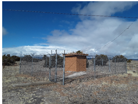
2021_ELMO_91760_El Morro Pump House_Front.jpg
