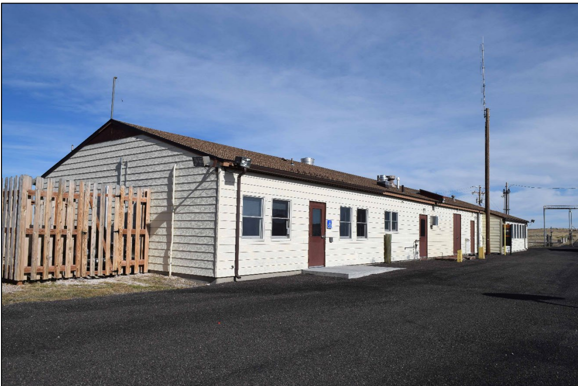
Photograph 16. LCSB front (south) wall (right) and west wall (left). View east.
