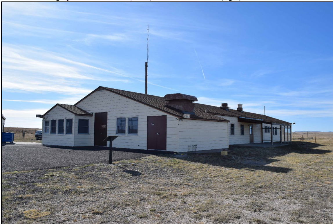
Photograph 18. LCSB rear (north) wall to right and east wall (left). View west-southwest.
