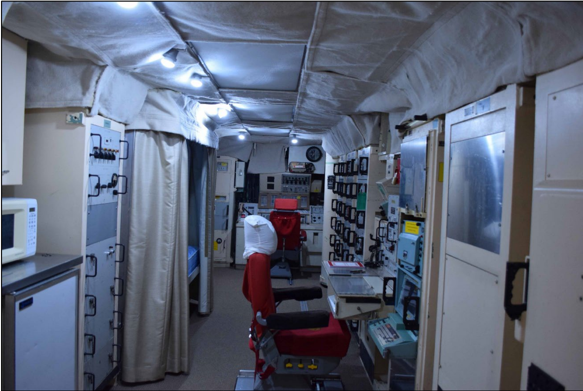
Photograph 7. Interior of the LCC from the north end. The commander's console is at the far end, the deputy commander's console is in the foreground to the right. Along the left wall are a microwave, refrigerator, and bunk. View south-southwest.
