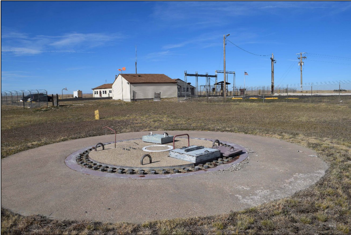
Photograph 25. Hardened high-frequency transmitting antenna. View north-northwest.
