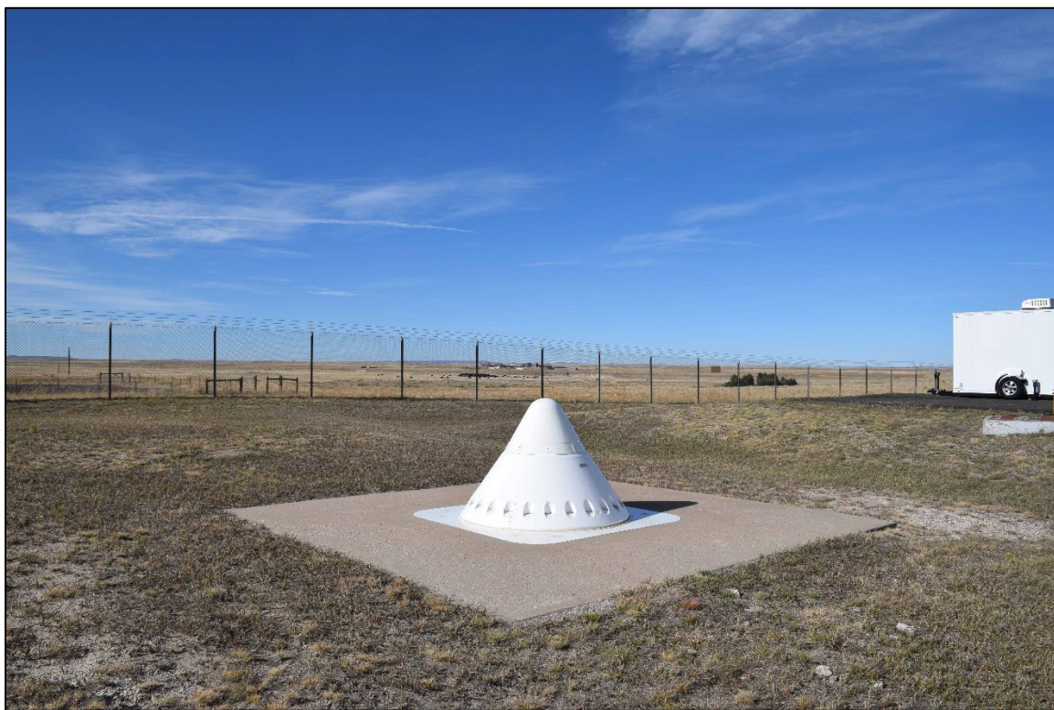
Photograph 24. Hardened ultra-high-frequency antenna. View north-northwest.
