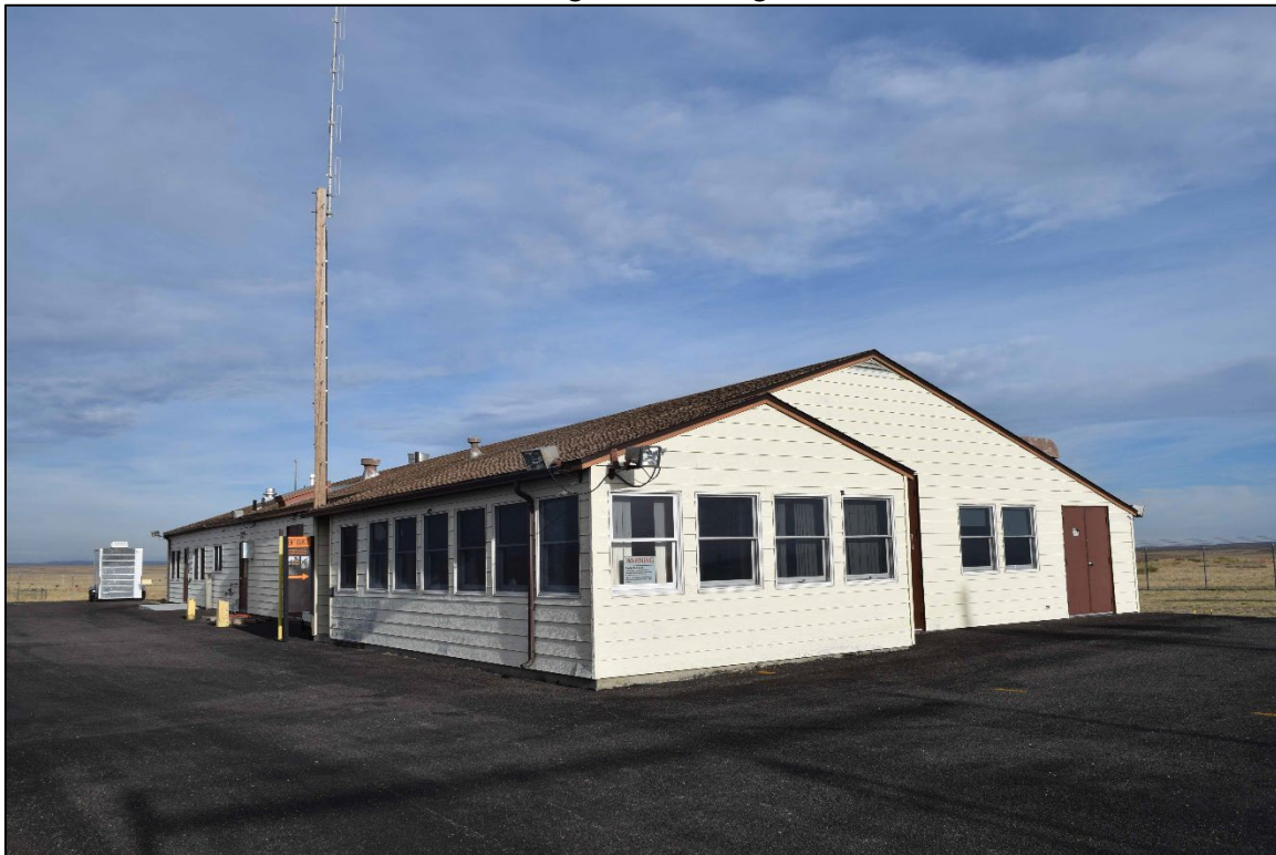
Photograph 14. Launch control support building (LCSB), front (south) wall (left) and east wall (right). View northwest.
