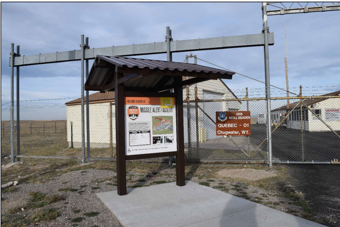
Photograph 30. Wyoming Parks information sign with the LCSB and vehicle storage building inside the security fence beyond. View west-northwest.
