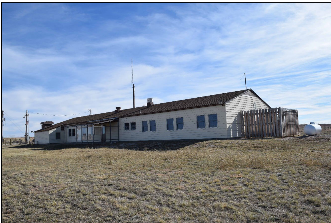
Photograph 17. LCSB rear (north) wall and west wall (right). View southeast.
