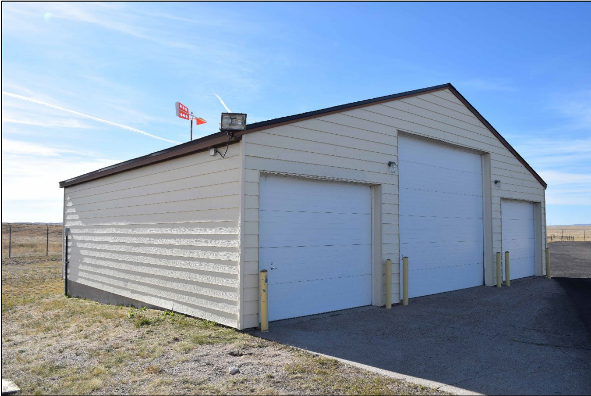
Photograph 21. Vehicle storage building, front (north) and east walls. View west.
