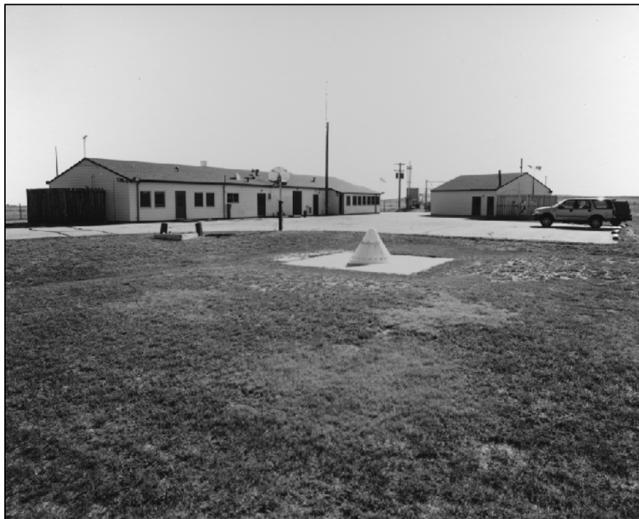
Figure 14. The launch control support building is to the left and the vehicle storage building stands at right in this 1999 photograph (view east). Courtesy of Historic American Engineering Record draft documentation, Photograph HAER WY-89, 1999.
