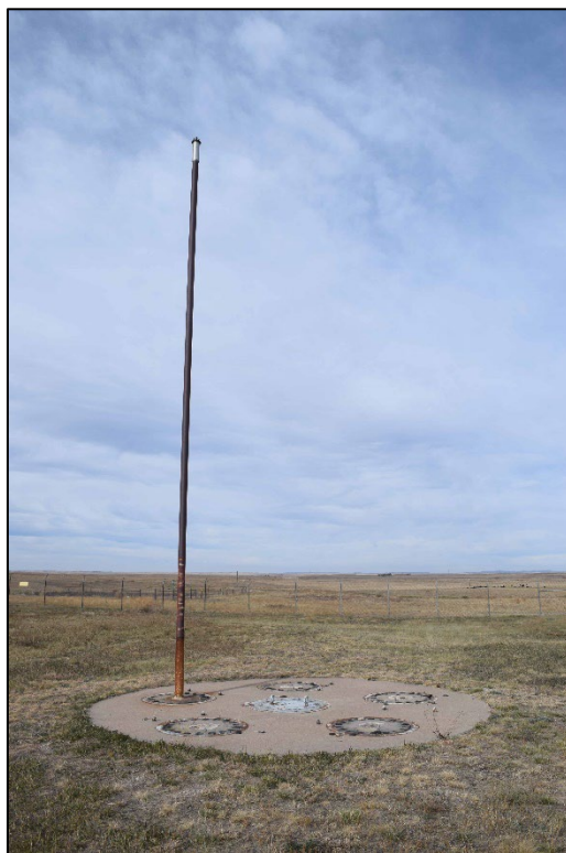
Photograph 23. Hardened high-frequency receiving antenna. View southwest.
