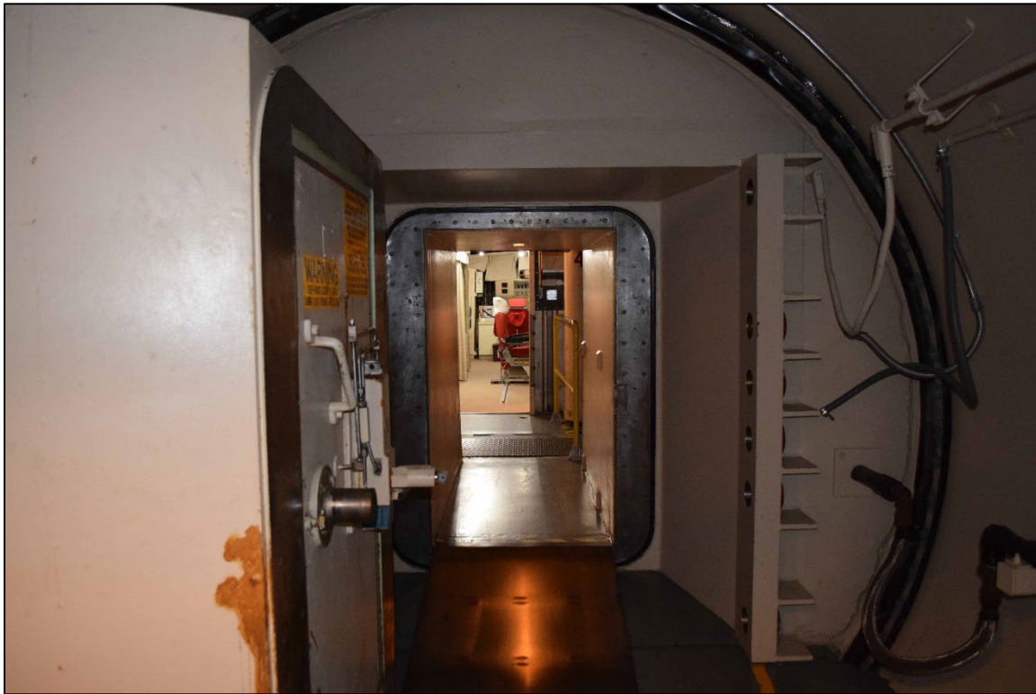
Photograph 5. View from tunnel junction into the LCC. The blast door is to the left. View south-southwest.
