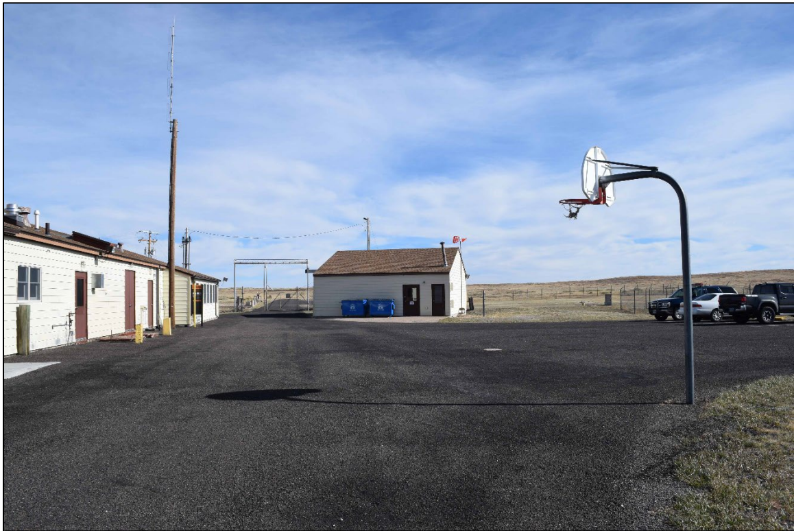
Photograph 3. Overview from west edge of parking area, showing launch control support building (left) and vehicle storage building and basketball pole to right. View east-southeast.
