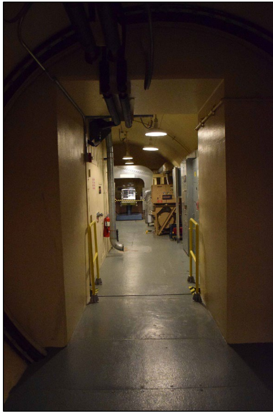
Photograph 11. View of the LCEB from the tunnel junction. View north-northeast.
