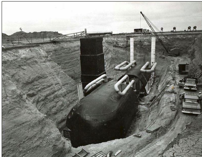
Figure 5. Subsurface construction was underway in 1963 at a similar launch control facility. The launch control center (LCC) is in the foreground with the elevator shaft to the left and the launch control equipment building (LCEB) in the background. The opening for the escape tube to the surface is at the top left of the near end of the LCC. The vertical white pipes are the air intake and exhaust ducts. Courtesy of 90 th Civil Engineering Squadron, F.E. Warren AFB, in Historic Structure Report, Missile Alert Facility Quebec-1 , 1-8.
