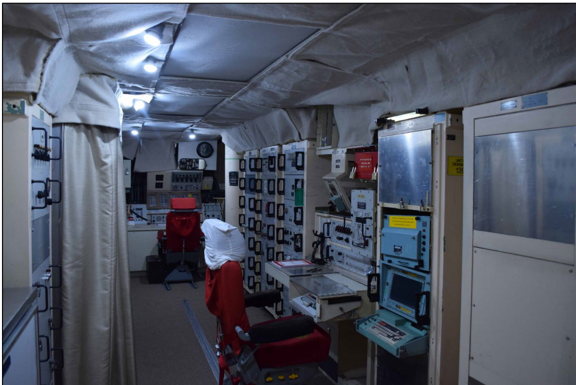
Photograph 10. The west wall of the LCC holds the DMCCC's console (right) and the south wall the MCCC's console (in distance to left). View southwest.
