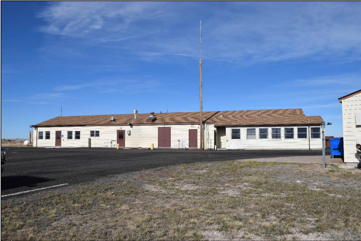
Photograph 15. LCSB front (south) wall, with vehicle equipment building to right. View north-northeast.
