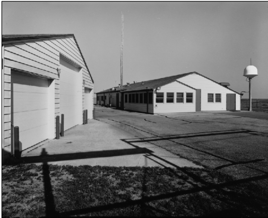
Figure 13. The launch control support building and ICBM super-high frequency satellite terminal (ISST) (the radome) stand to the right and vehicle storage building is at left in this 1999 photograph (view northwest). Courtesy of Historic American Engineering Record draft documentation, Photograph HAER WY-89-006, 1999.
