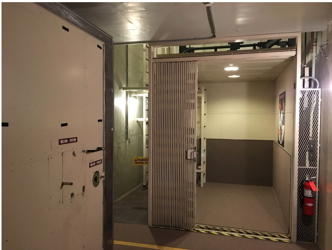
Photograph 4. View of freight elevator from the tunnel junction. View east-southeast.
