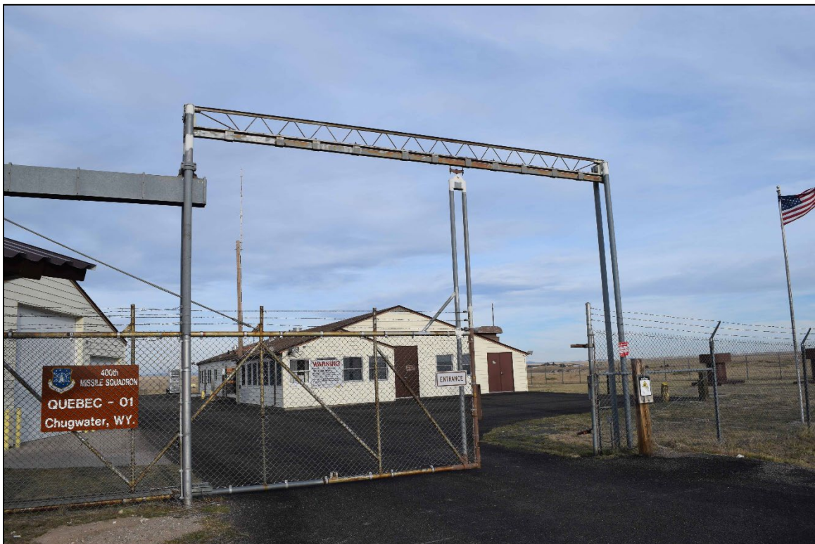
Photograph 2. Security gate with the launch control support building, flagpole, and air intake and exhaust ducts to right and vehicle storage building to left. View northwest.
