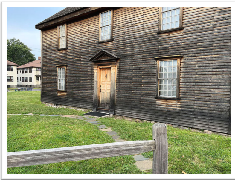
Figure 2 – Universal Accessibility: Showing existing conditions of stepping-stone pathways, John Adams house.
