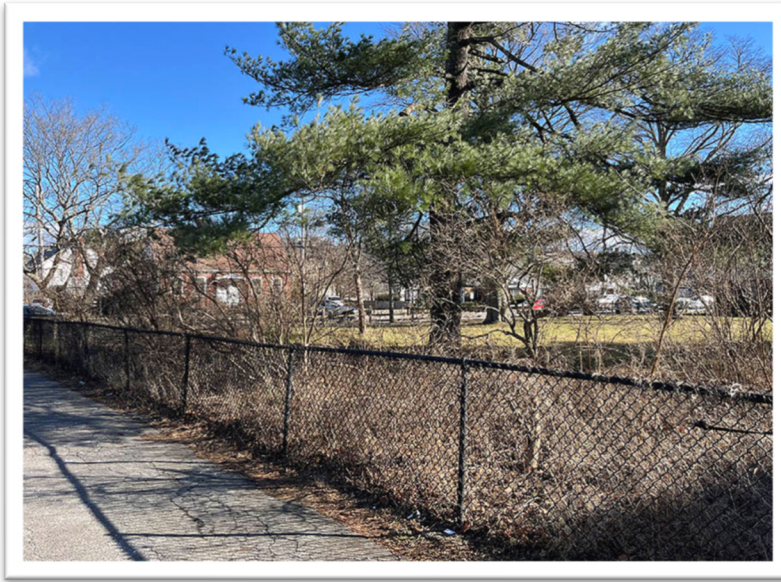
Figure 12 – Existing fencing to be replaced with stockade fencing at the Northern Site Boundary. Photo taken from off-site, within adjacent commercial parking lot.
