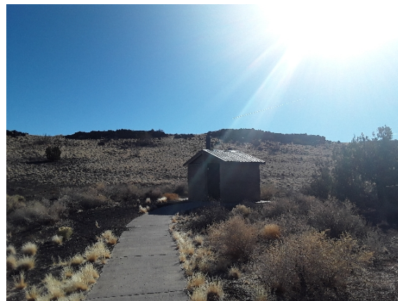
2020_WUPA_48508_WUPA Lomaki Restroom_Z.jpg
