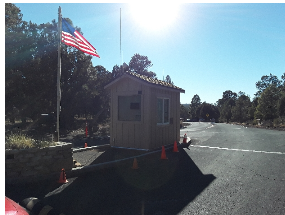
2020_WACA_51280_WACA Entrance Station_P_.jpg
