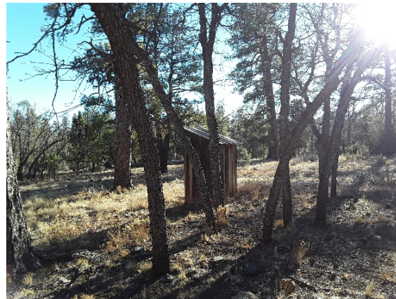
2020_WACA_46819_WACA CCC Restroom_Z.jpg
