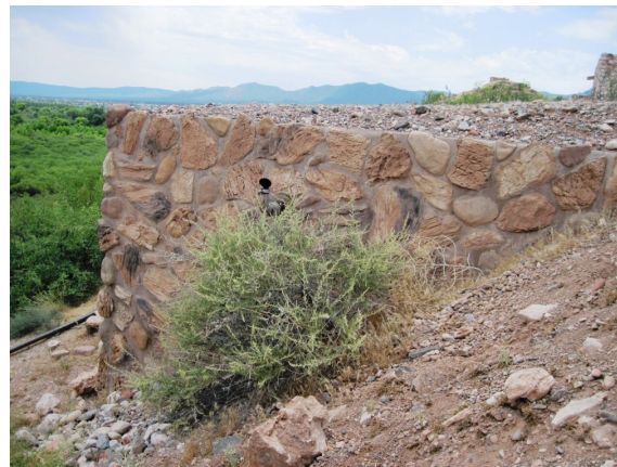
2018_TUZI_74442_Fire Pump Building_D.jpg
