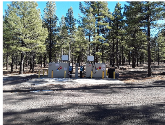
2020_SUCR_Not found_Fuel Pumps / Tanks_Front.jpg
