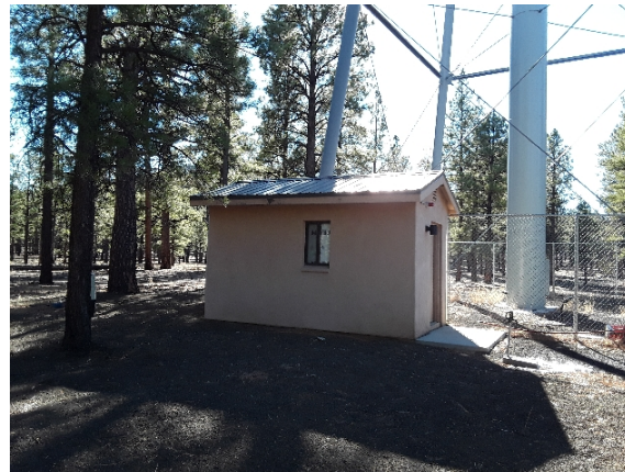
2020_SUCR_48439_SUCR Pump House Building_Z.jpg
