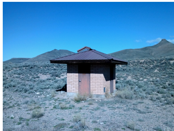
CURE_75019_Stevens Creek Pumphouse_Front.jpg
