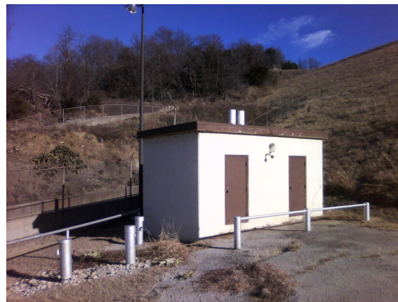
CHIC__Dam Control Building_Front.jpg
