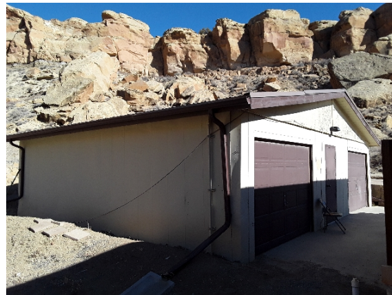
2021_CHCU_71973_Lumber Storage Shop_Front.jpg
