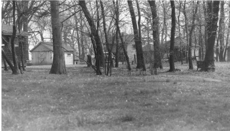
The Domestic Service Cluster in ca. 1931, looking southeast through woods. (Image Credit: National Park Service)
