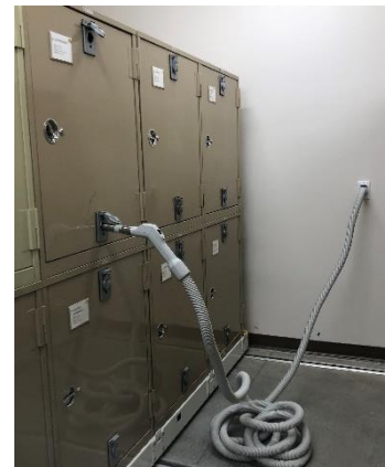
Image 1: Former vacuum port system with top port open to prevent pressure buildup.
