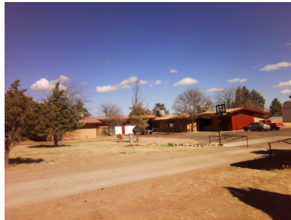
FODA_55218_Housing Office Triplex MA.jpg
