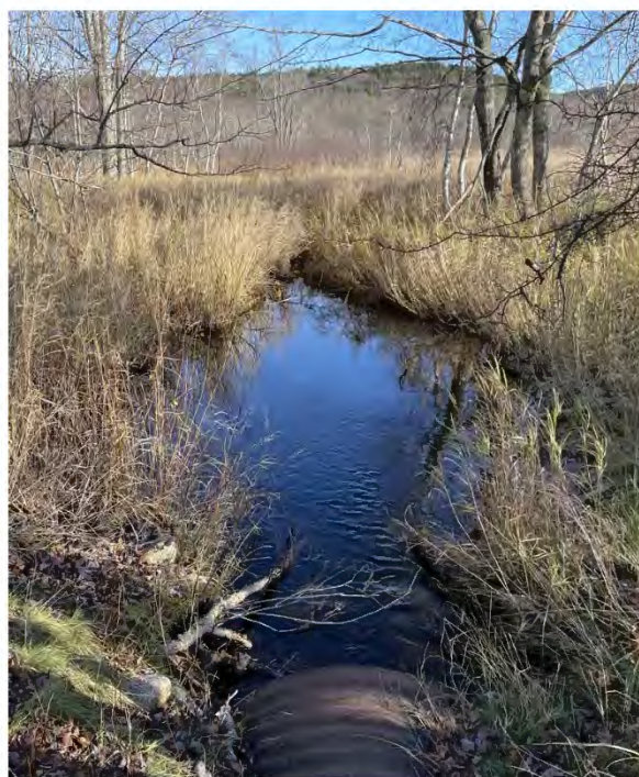
Photo 16: Culvert under Hemlock Path (Hemlock-8). Hemlock Path splits the wetland to the west from the Great Meadow, concentrating flow through this culvert.
