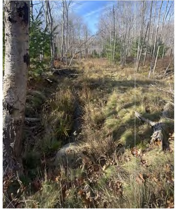
Photo 4: Culvert under Park Loop Road (Park Loop Rd-6). An old roadbed within this watershed collects and concentrates flow from upland areas, causing erosion downstream.
