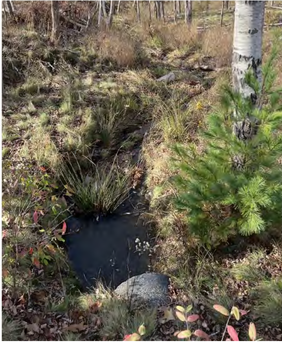
Photo 3: Culvert under Park Loop Road (Park Loop Rd-5). Channel erosion observed downstream from concentrated flow at culvert.
