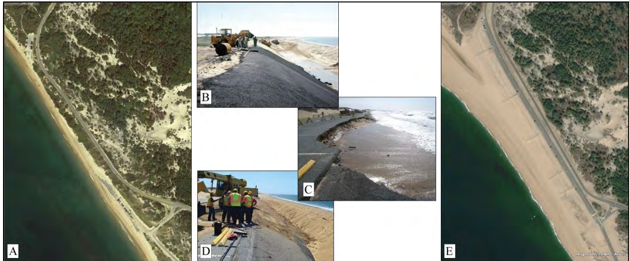
Figure 3. A and E: Images of Herring Cove Beach, Provincetown, MA, USA before (2018) and after (2021) the parking lot was moved ~80 m landward. Middle upper (B): Image of asphalt being placed on sand from the 1960s at Herring Cove Beach. Middle Center (C): 2017 coastal erosion undermining parking lot at Herring Cove. This was one of several repaving projects from 2010-2018. Middle Bottom (D): Seashore crew repairing parking lot, circa 2015.
