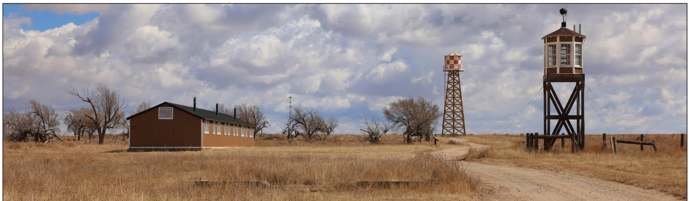
Barracks, water tower, and guard tower (from left to right), at Amache NHS, located in Granada, Colorado. Japanese Americans were incarcerated at the site from 1942-1945, during World War II. NPS Photo.
