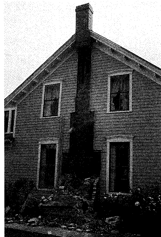
Historic Preservation Partners for Earthquake Response funded a study that provided alternative engineering and design guidelines that met current building codes for chimney repair and restoration.
