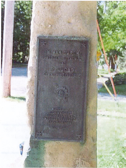
Figure 8. Plaque added to monument by Daughters of the American Revolution in 1935. Photo shows copper staining, which has leached out from the bronze and deeply stained the limestone along the water runoff channel. June 2017.
