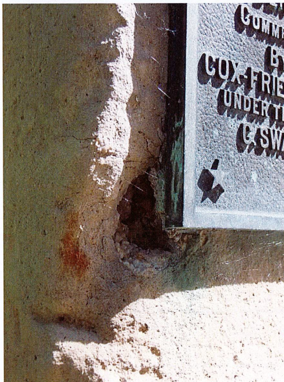
Figure 11. Damage to monument where plaques were attached. June 2017.
