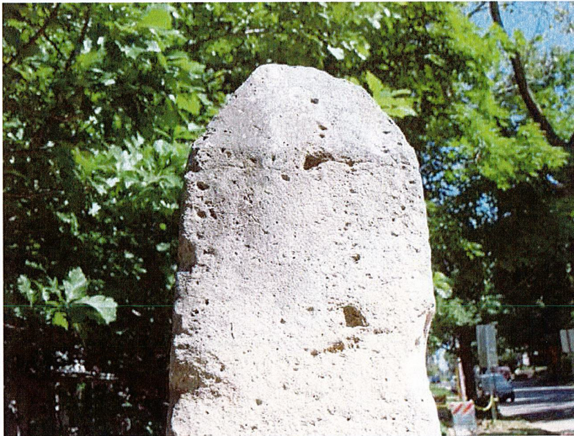
Figure 10. The limestone of the monument is weathered and deteriorating. June 2017.
