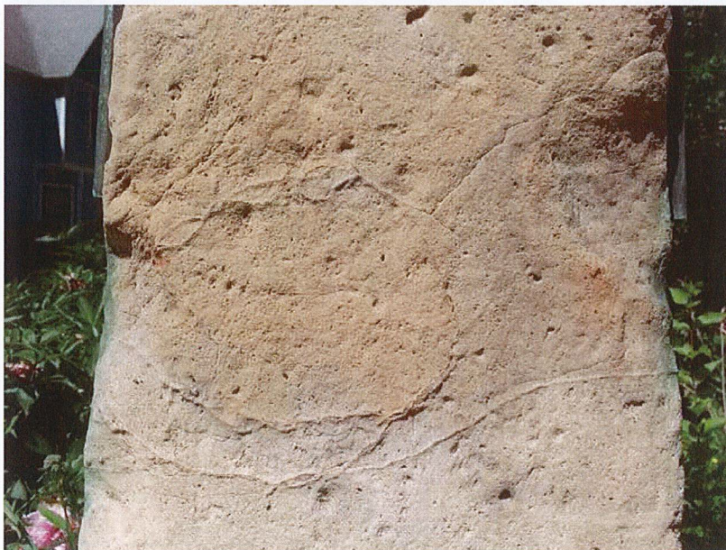
Figure 13. Uneven weathering and wear patterns attributed to the specific geology and formation of limestone which is composed of layers of compressed sand and shell fragments cemented together with mineral binders, primarily calcite crystals. June 2017.
