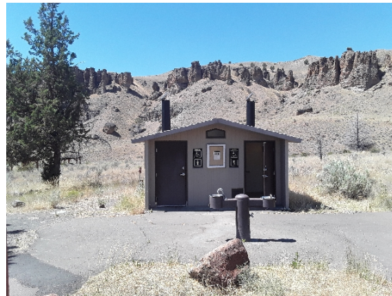
2022_JODA_88261_CL BLDG Restrooms_Front.jpg
