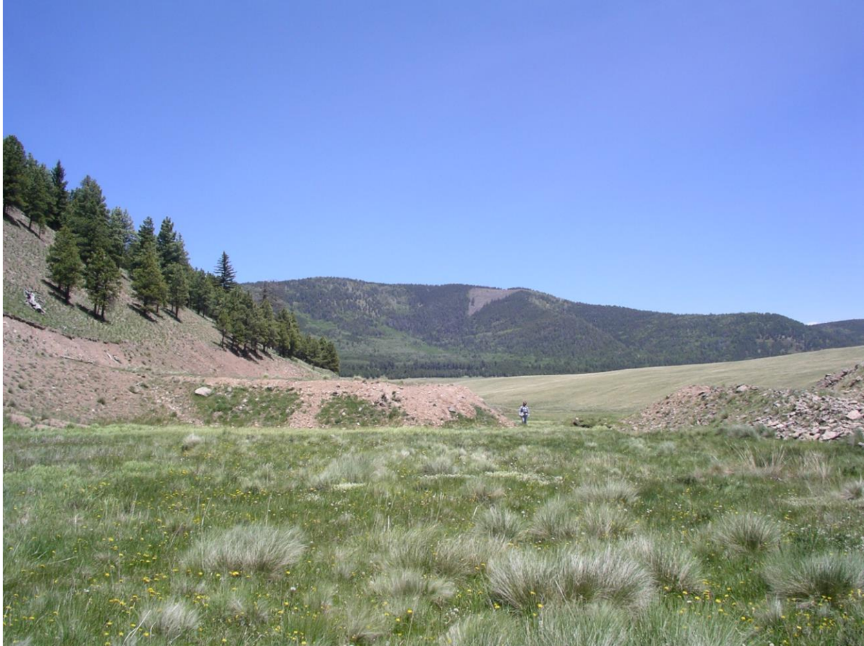
Photo 11: Reach 1, NSO 46 R23, looking upstream at non-functioning, historic dam with Z. Manickam streamside (6-June-2007).
