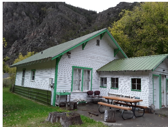
2022_BLCA_not found_Caretakers Residence_Front.jpg
