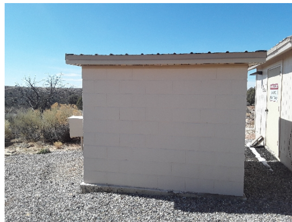
2020_HOVE_61481_Old Pump House_Front.jpg
