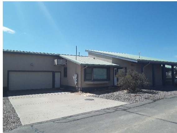
2020_HOVE_81575_H-9 Duplex (Housing # 4)_Front.jpg
