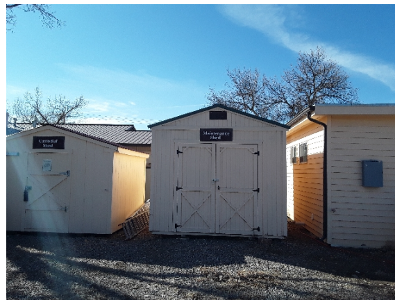
2021_AZRU_not found _Maintenance Shed_Front.jpg
