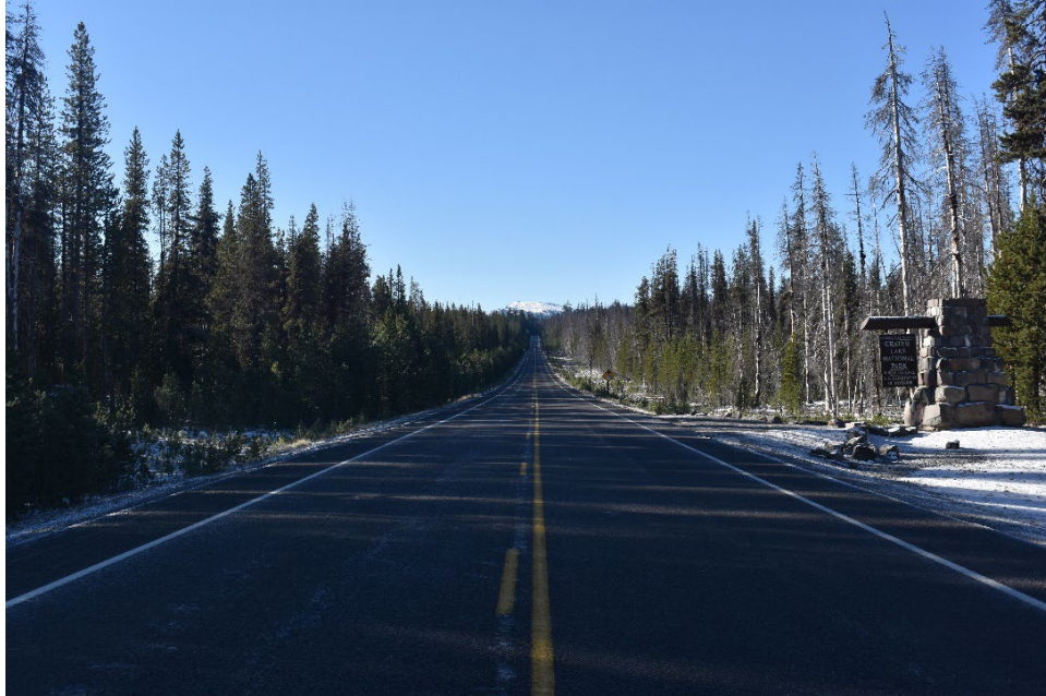
Photograph 1. Overview North Entrance Road at the North Entrance boundary, facing north, October 12, 2021. (OR_Klamath County and Douglas County_North Entrance Road_001)
