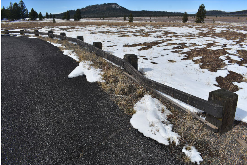
Photograph 26. Overview Pumice Desert Wayside Exhibit guardrail detail, view facing west, October 12, 2021. (OR_Klamath County and Douglas County_North Entrance Road_026)
