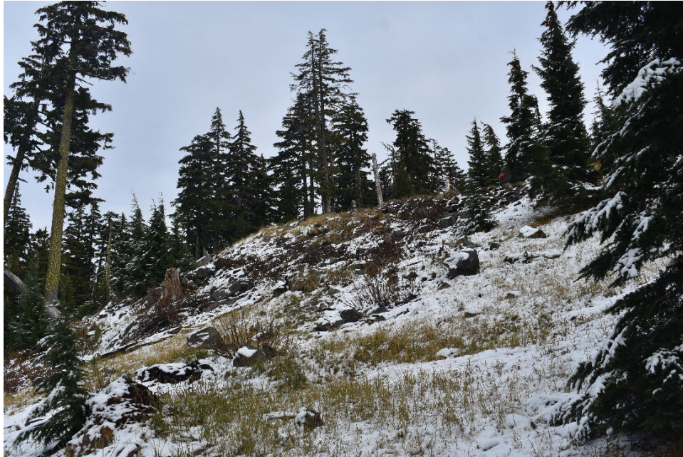
Photograph 13. Overview of the remnants of a retaining wall, approaching the North Junction beneath the Blowdown Pullout, view facing east, October 12, 2021. (OR_Klamath County and Douglas County_North Entrance Road_013)
