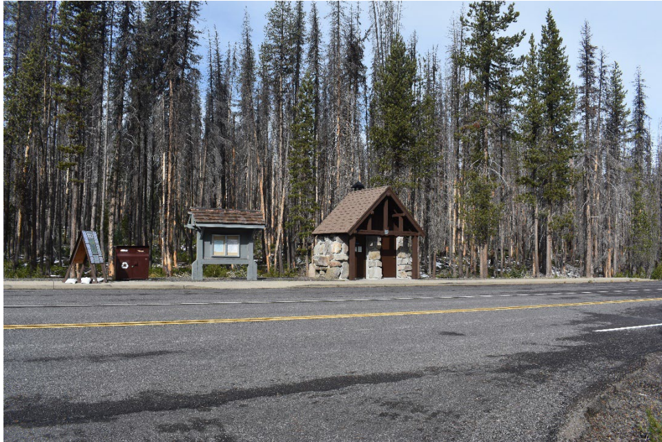
Photograph 9. Overview of the North Entrance Kiosk pullout, view facing northwest, October 12, 2021. (OR_Klamath County and Douglas County_North Entrance Road_009)
