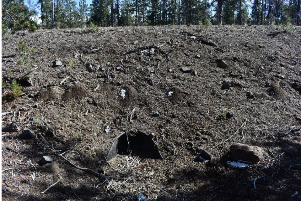
Photograph 21. Culvert on the west side of the North Entrance Road, located south of the Pumice Desert Wayside Exhibit, October 12, 2021. (OR_Klamath County and Douglas County_North Entrance Road_021)
