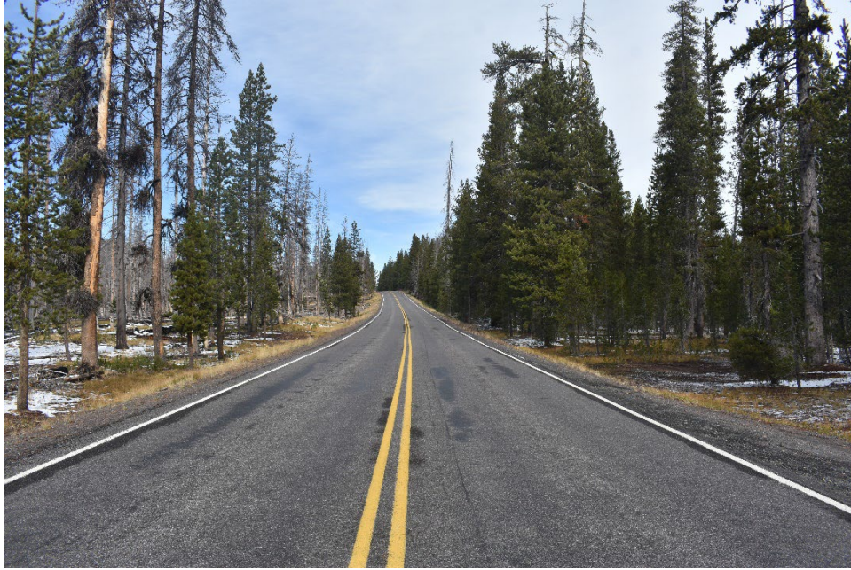
Photograph 5. Overview of vegetation and road, located north of the Pumice Desert, view facing north, October 12, 2021. (OR_Klamath County and Douglas County_North Entrance Road_005).
