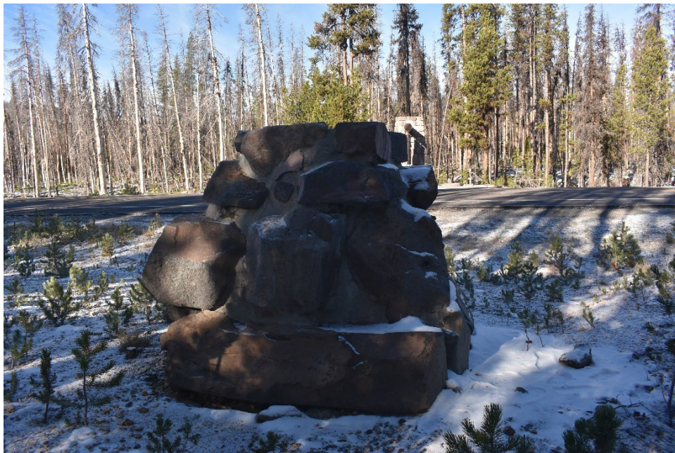
Photograph 4. North Entrance bollards, facing south, October 12, 2021. (OR_Klamath County and Douglas County_North Entrance Road_004)
