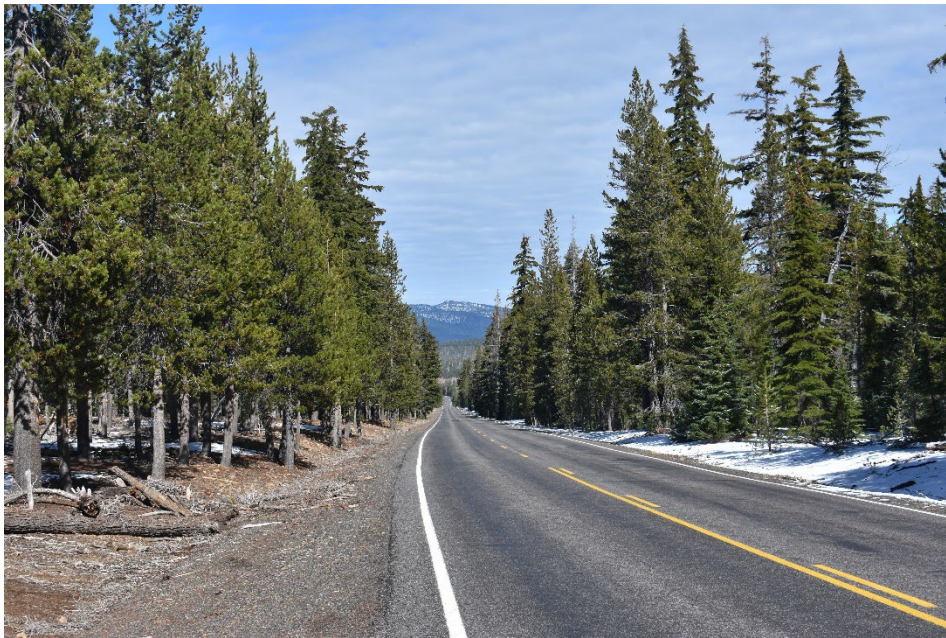
Photograph 7. Overview of road alignment, located north of the Pacific Crest Trail parking area, view facing north, October 12, 2021. (OR_Klamath County and Douglas County_North Entrance Road_007)
