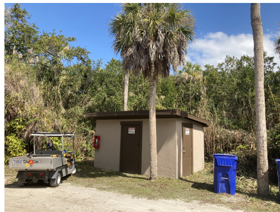
2022_DESO_75317_Fuel and Paint Shed_Front.jpg
