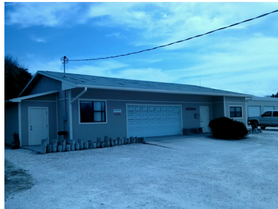
2017_CANA_60158_ND Maintenance Shop_Front. jpg
