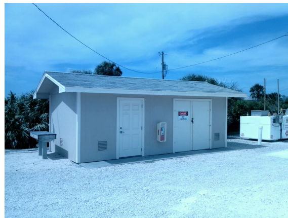
2017_CANA_60162_ND P.O.L. Building_Front.jpg
