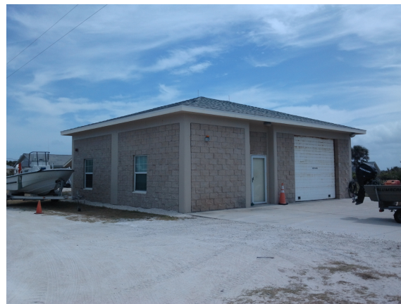
2017_CANA_99410_ND Fire Cache Building_Front.jpg
