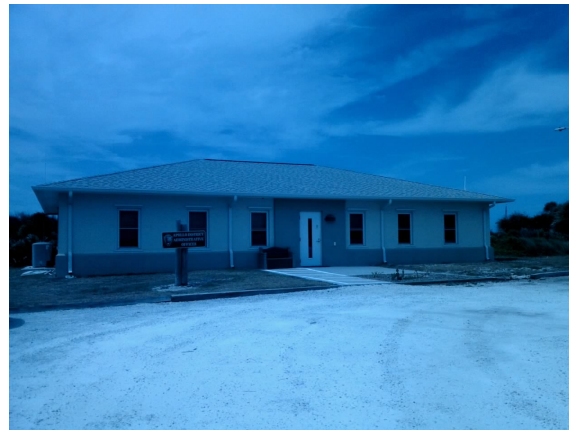
2017_CANA__Apollo District Admin Offices_Front. jpg
