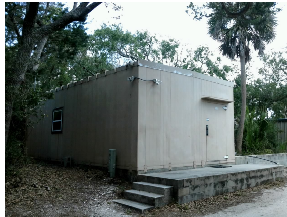
2017_CASA_37049_FOMA Balley Building_Front.jpg
