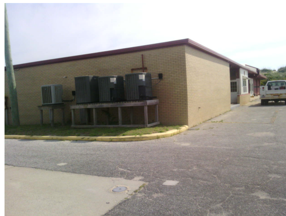
2016_CAHA_28888_BI BD Maintenance Shop_Front.jpg
