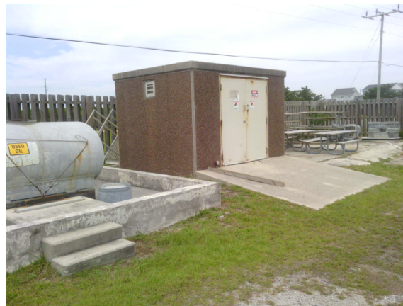
2016_CAHA_28909_BI BD Haz-Mat Building_Front.jpg
