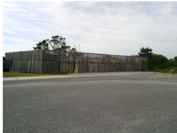
2016_CAHA__oregon fishing center fuel tanks._Front.jpg
