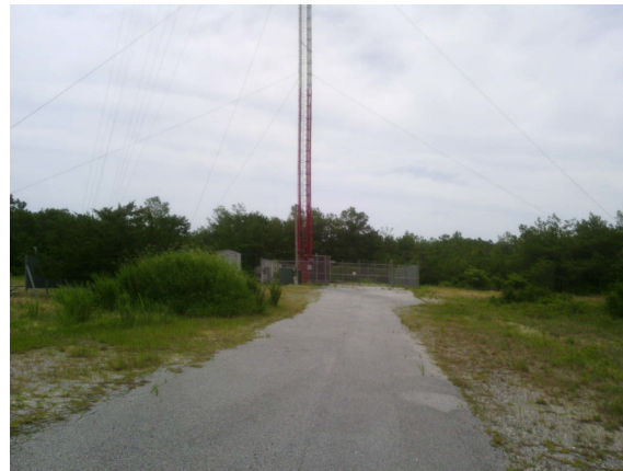
2016_CAHA__US Communication tower site_Front.jpg
