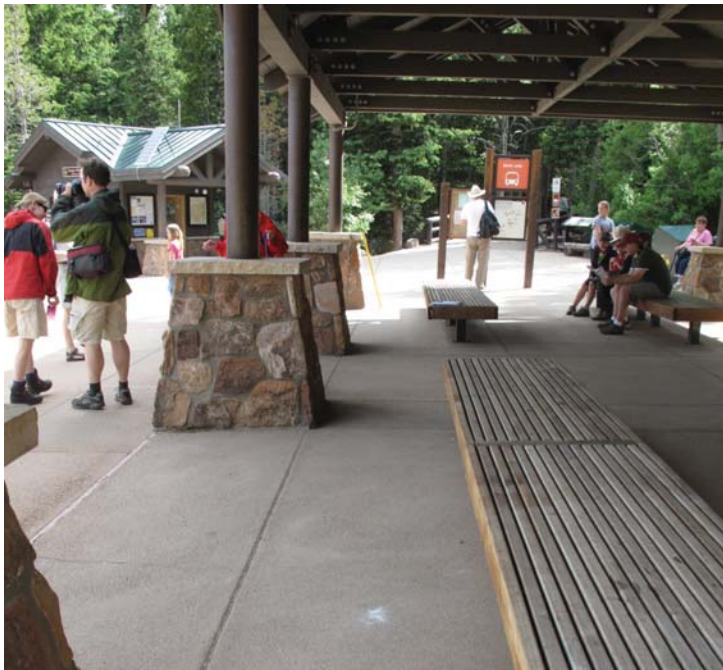
Bear Lake Bus Shelter in the Subalpine Zone
