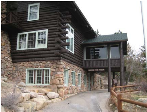
New and old construction in Rocky Mountain National Park that creates a unified design experience while using sustainable building methods.
