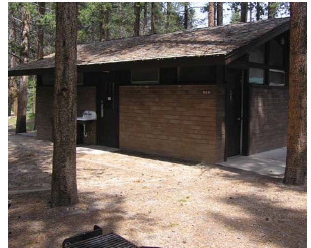
Notice pre-fabricated materials including brick wall. Example of Mission 66 Comfort Station in Timber Creek Campground c. 1963.
