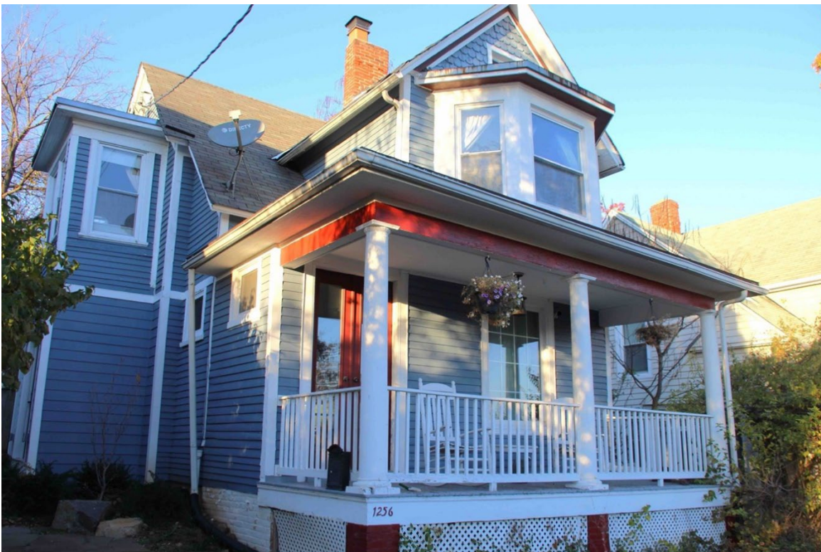
Photo 4 (DC_Slowe Burrill House_0004)
