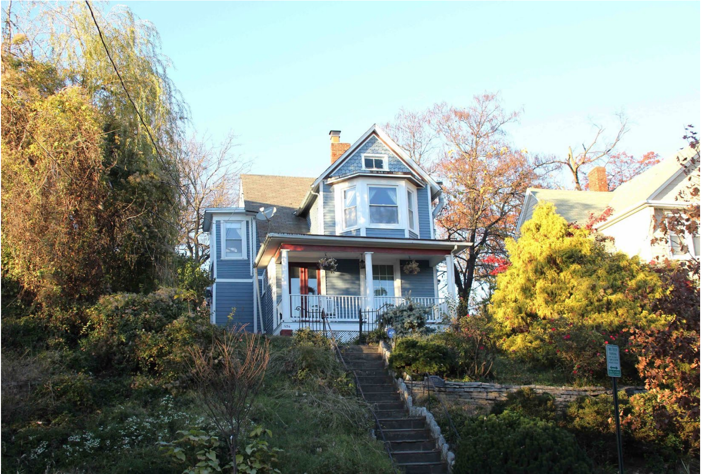
Photo 1 (DC_Slowe Burrill House_0001)
