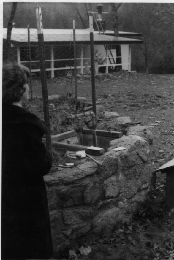
WHIS WR # 9 - Strombeck Well Well is located in small pit in flower garden. Well provides domestic supply for NPS residences # 86 & 78. Werrell Jan 14, 1976
