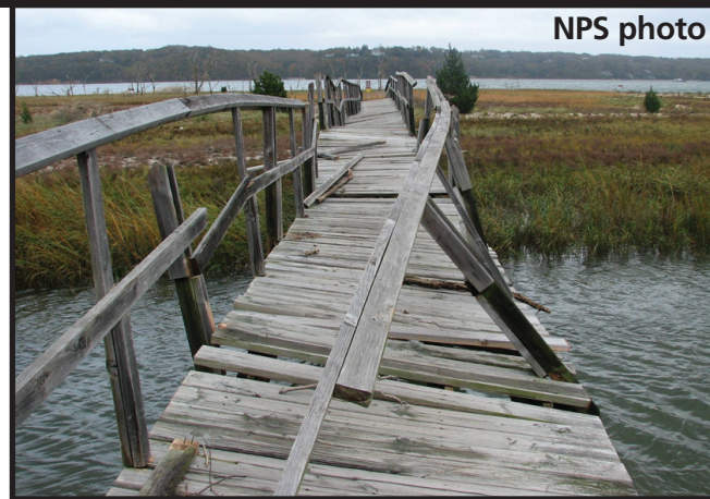
Damage to the nature trail boardwalk following Hurricane Sandy in October 2012
