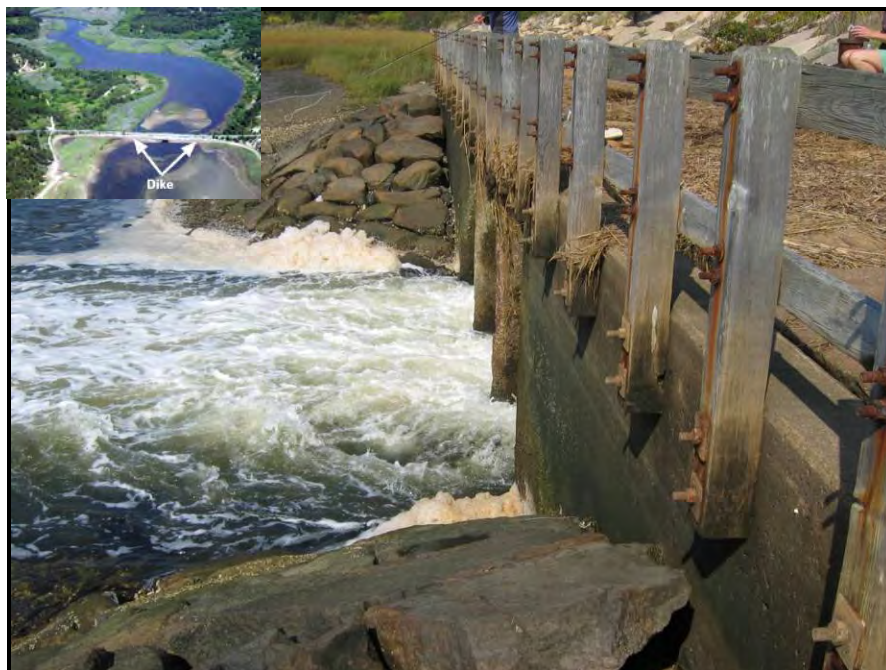
Figure 1-2. Dike structure at the Chequessett Neck Road crossing.
