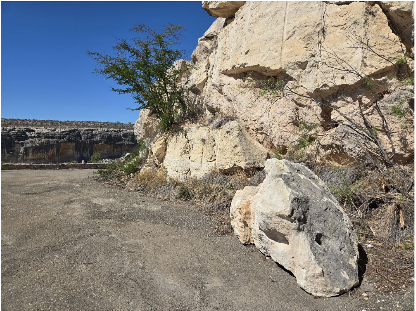
Figure 22. Photograph of a rockfall at the Pecos River boat ramp. Rockfalls are a common phenomenon along the steep cliffs flanking the river corridors in AMIS. NPS photograph/J. Johnson.
