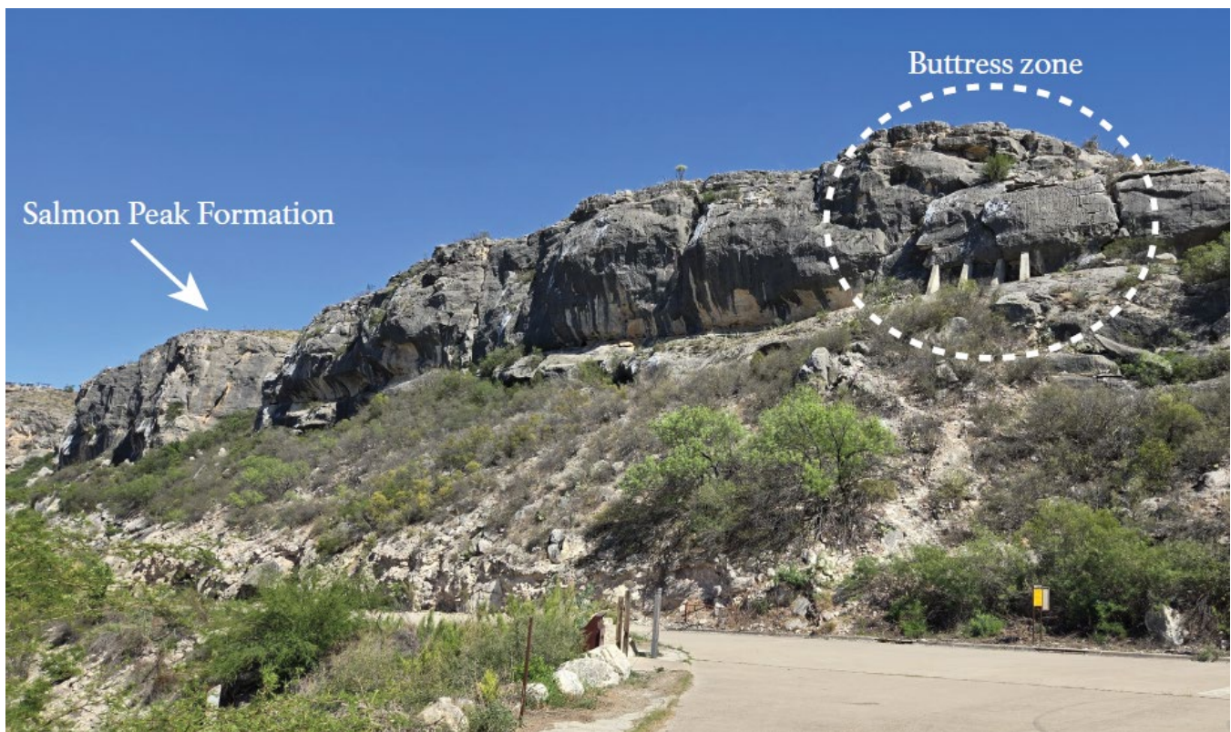
Figure 23. A massive limestone block supported by cement buttresses at the Pecos River boat ramp. Following a failed removal attempt by engineers, a large unstable block of the Salmon Peak Formation was supported using concrete buttresses (circled). NPS photograph/J. Johnson.
