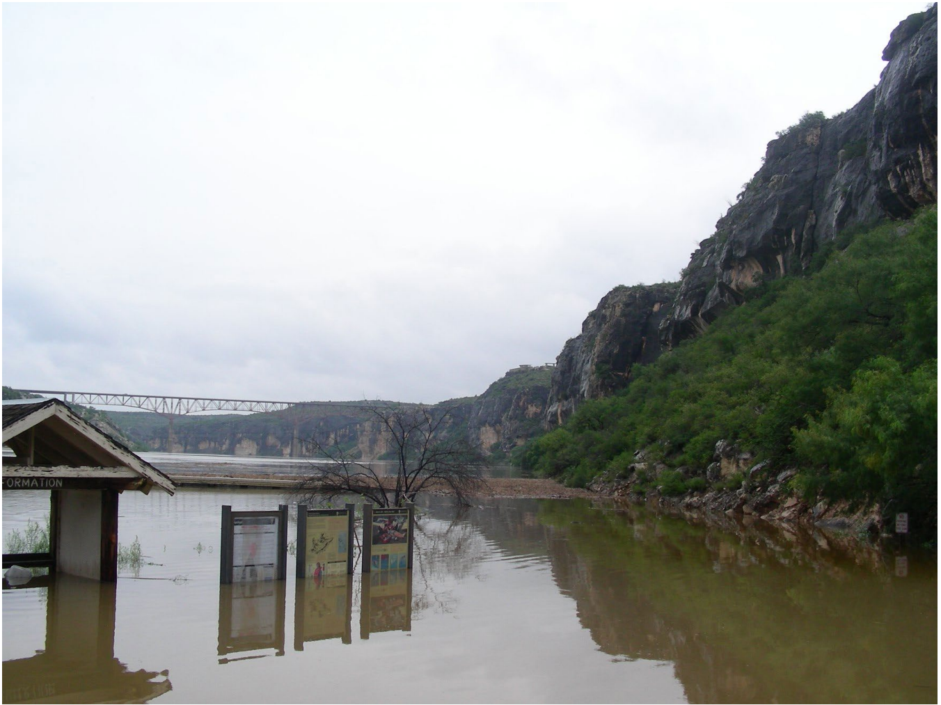
Figure 20. Photograph of flood conditions along the Pecos River in 2010. View is facing upstream (east) toward the US Highway 90 bridge. The Pecos River flood stage has overwhelmed the floodplain, including the boat ramp and other infrastructure. NPS photograph.
