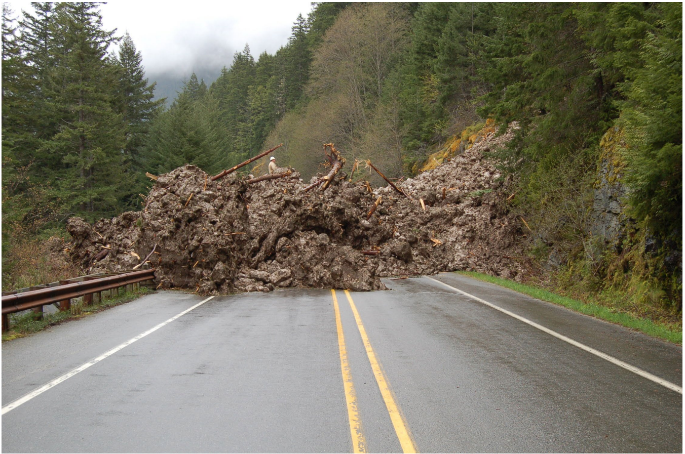
Figure 7. Photograph of debris from a snow avalanche obstructing the North Cascades Highway in ROLA. Consisting of a chaotic mix of snow, rock, and woody debris, this 2011 avalanche originated from Ruby Mountain and blocked the highway near Lillian Creek. A roadway worker stands atop the avalanche for scale. NPS photograph.
