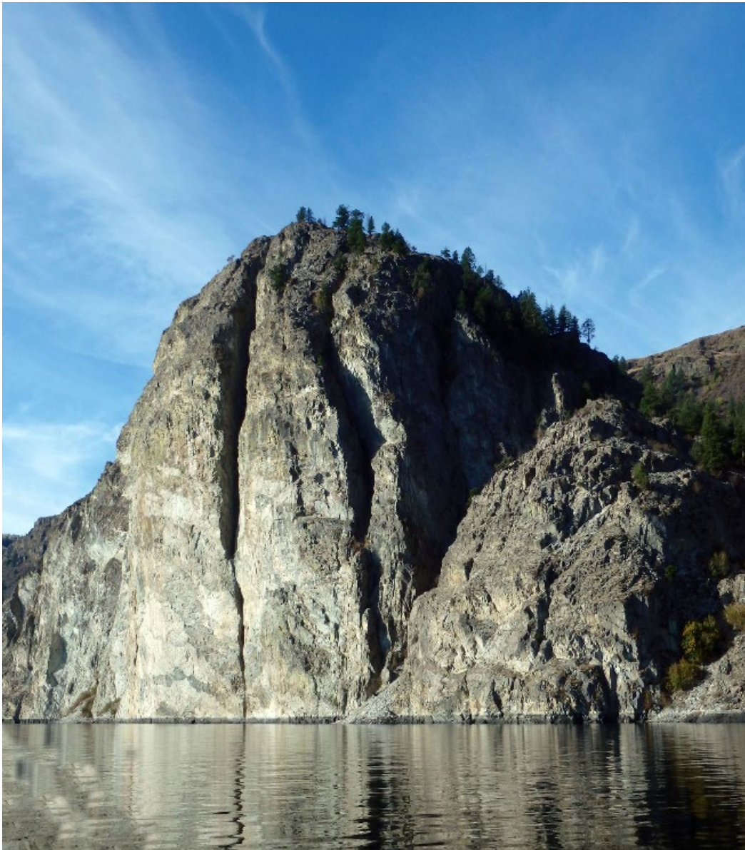
Figure 10. A view of Whitestone Rock along the south shore of Lake Roosevelt. Standing nearly 183 m (600 ft) above the surface of the reservoir, Whitestone Rock consists of Eocene intrusive rocks that are vertically fractured along its eastern face. These fractures facilitate exfoliation and bedrock landslides. NPS photograph.
