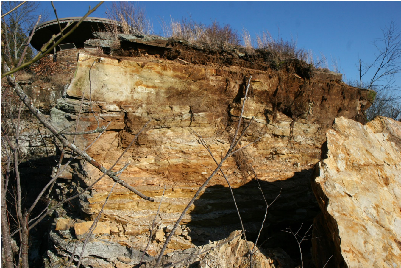
Figure 12. Photograph of the rockslide, taken in 2010, showing the bedrock underlying the eastern overlook. The rocks consist of sandstone and siltstone of the Wedington Sandstone Member of the Fayetteville Shale. NPS photograph.
