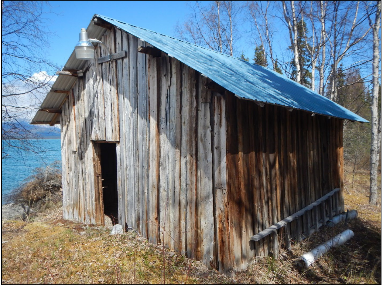
Photograph 3: Charlie Wolff Smokehouse, Toward North, NPS Historic Structure Inventory Program, 2024
