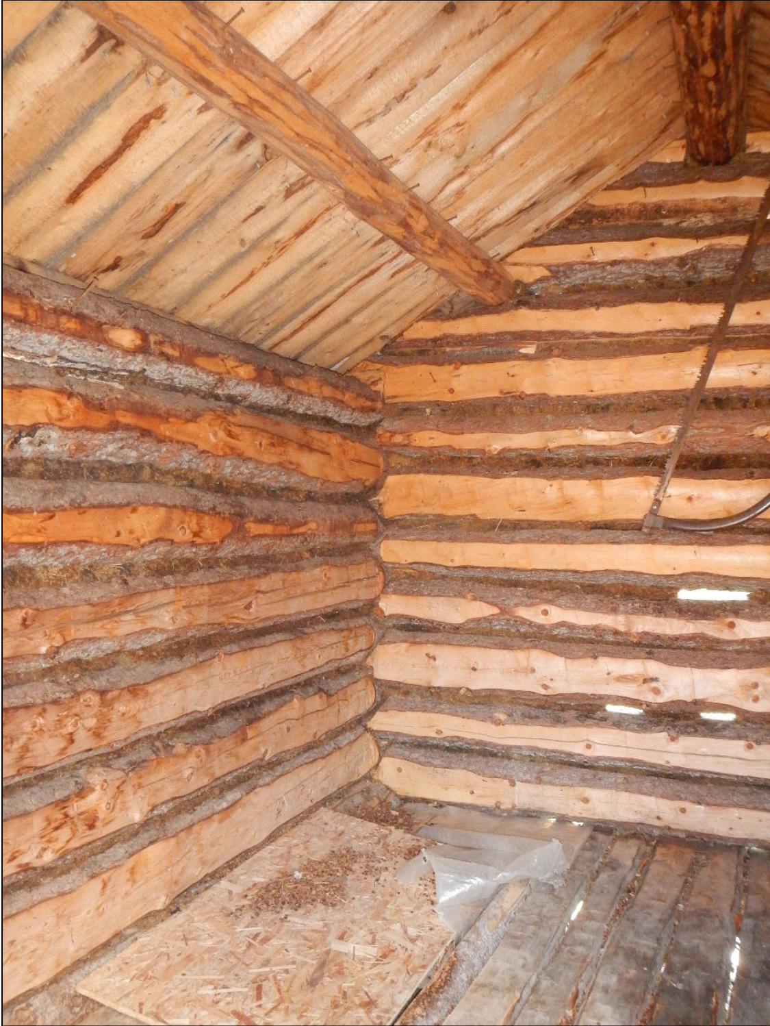
Photograph 9: Interior of Charlie Wolff Cache, NPS Historic Structure Inventory Program, 2024
