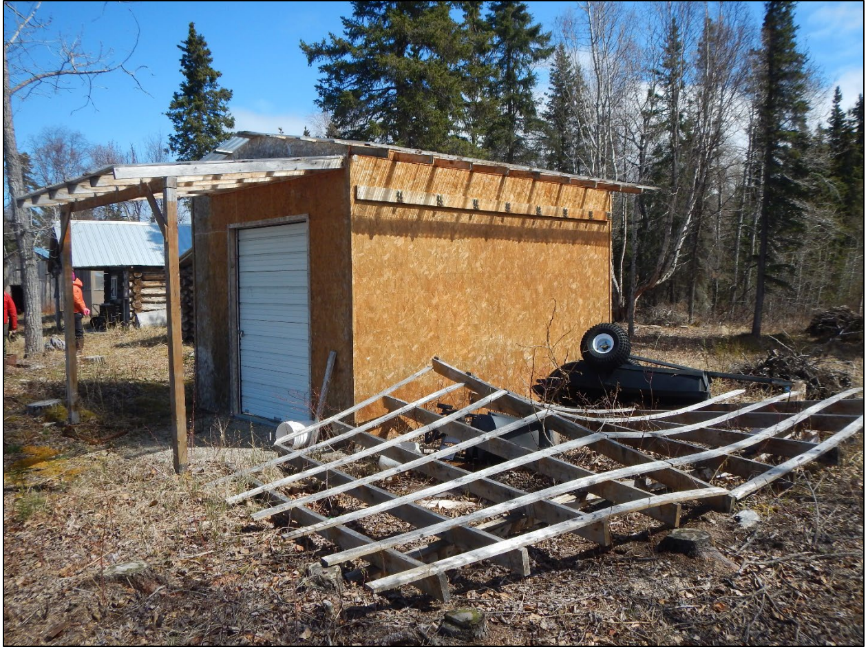
Photograph 7: Hansen Garage, Toward Northeast, NPS Historic Structure Inventory Program, 2024
