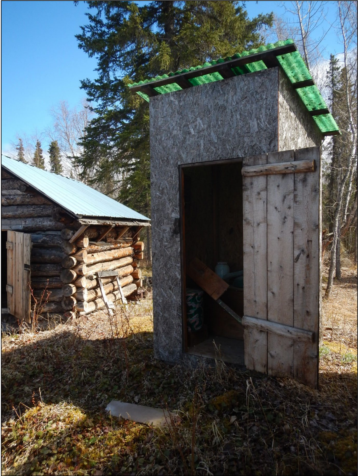
Photograph 6: Hansen Outhouse, Toward South, NPS Historic Structure Inventory Program, 2024
