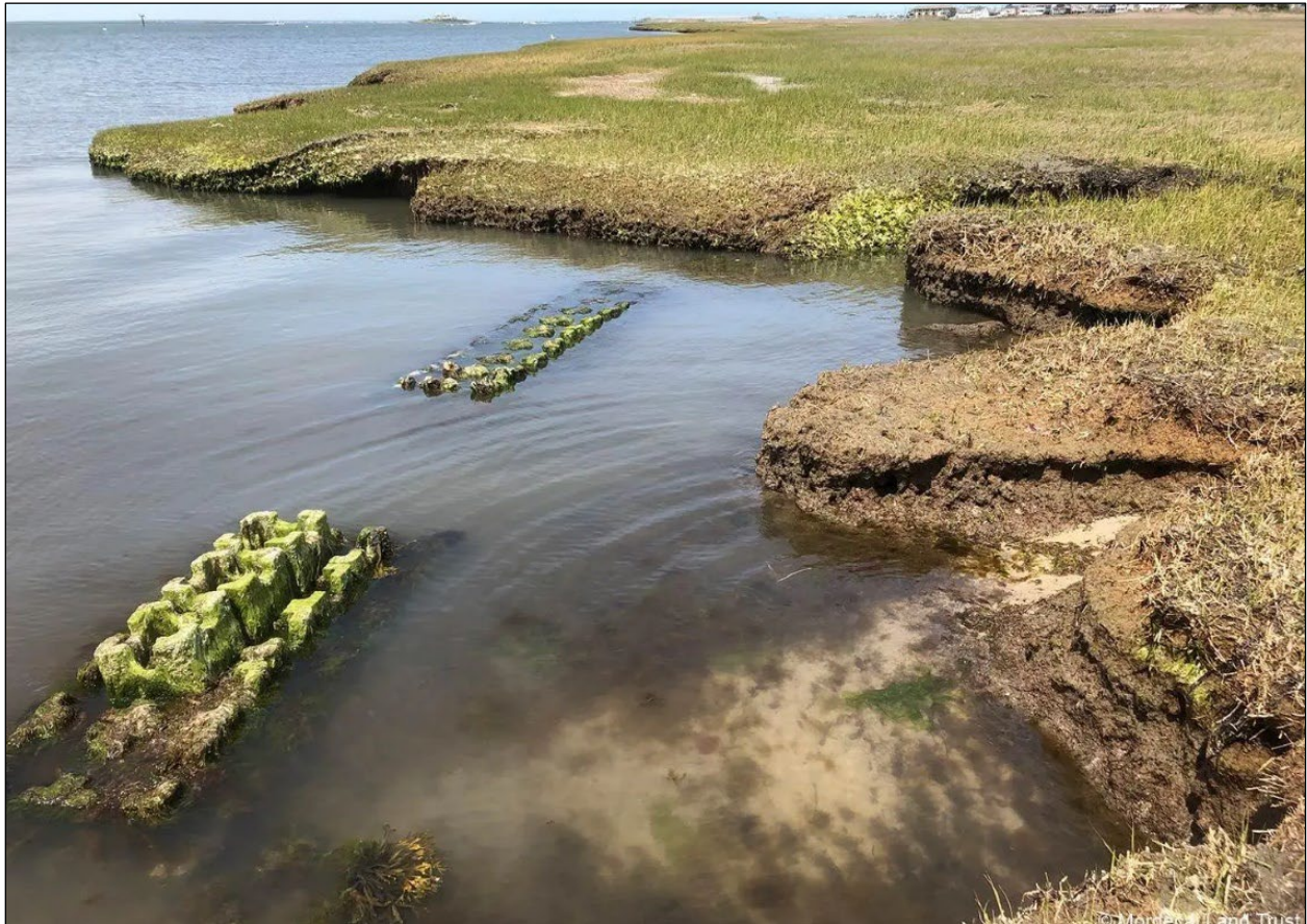
Figure 15 – An example of continuous lines of Wave Attenuation Devices deployed offshore to mitigate erosion at an Audubon site in Florida, from Living Shoreline Solutions ( livingshorelinesolutions.com , 2022).
