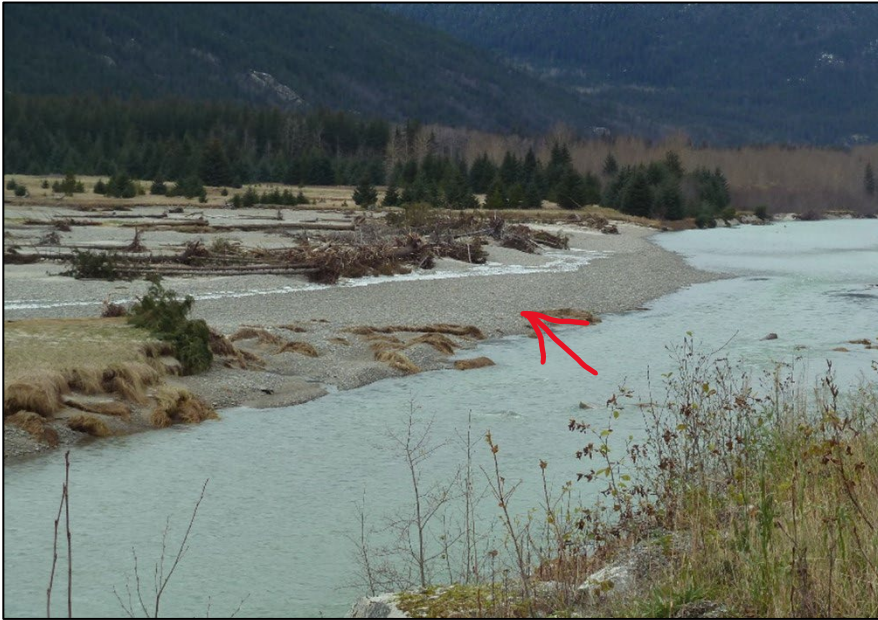
Arrow points to berm formation at former upstream opening to meander.
