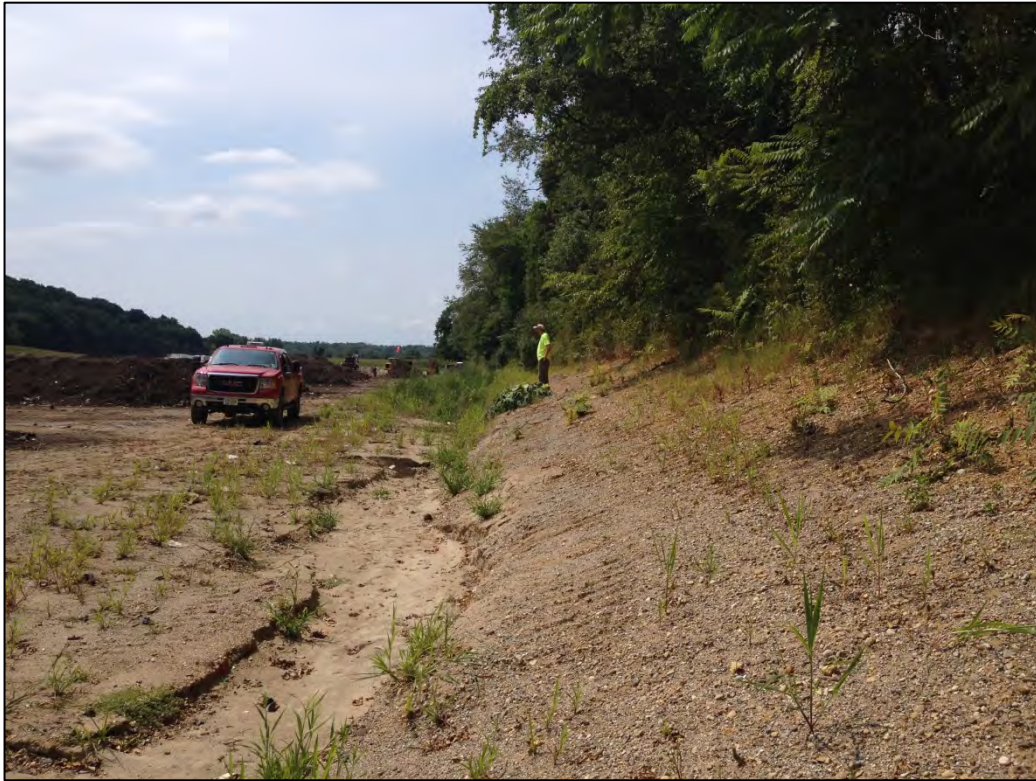
Photo 25: Drainage swale along perimeter of AgChoice stockyard.
