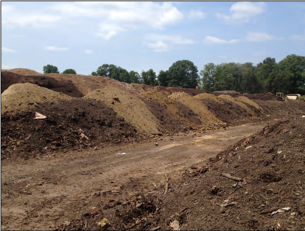
Photo 23: Staging for mixing of mineral (sand) and compost for final topsoil product at the AgChoice stockyard.
