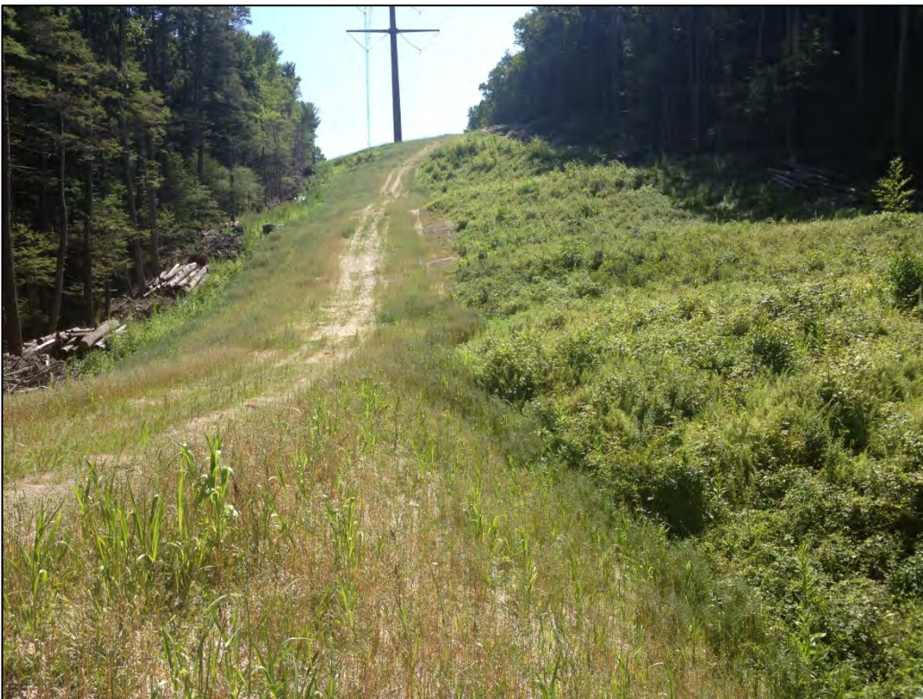
Photo 2: Access road between transmission structures showing restored, post-construction area (left) and un-impacted, un-restored area (right).
