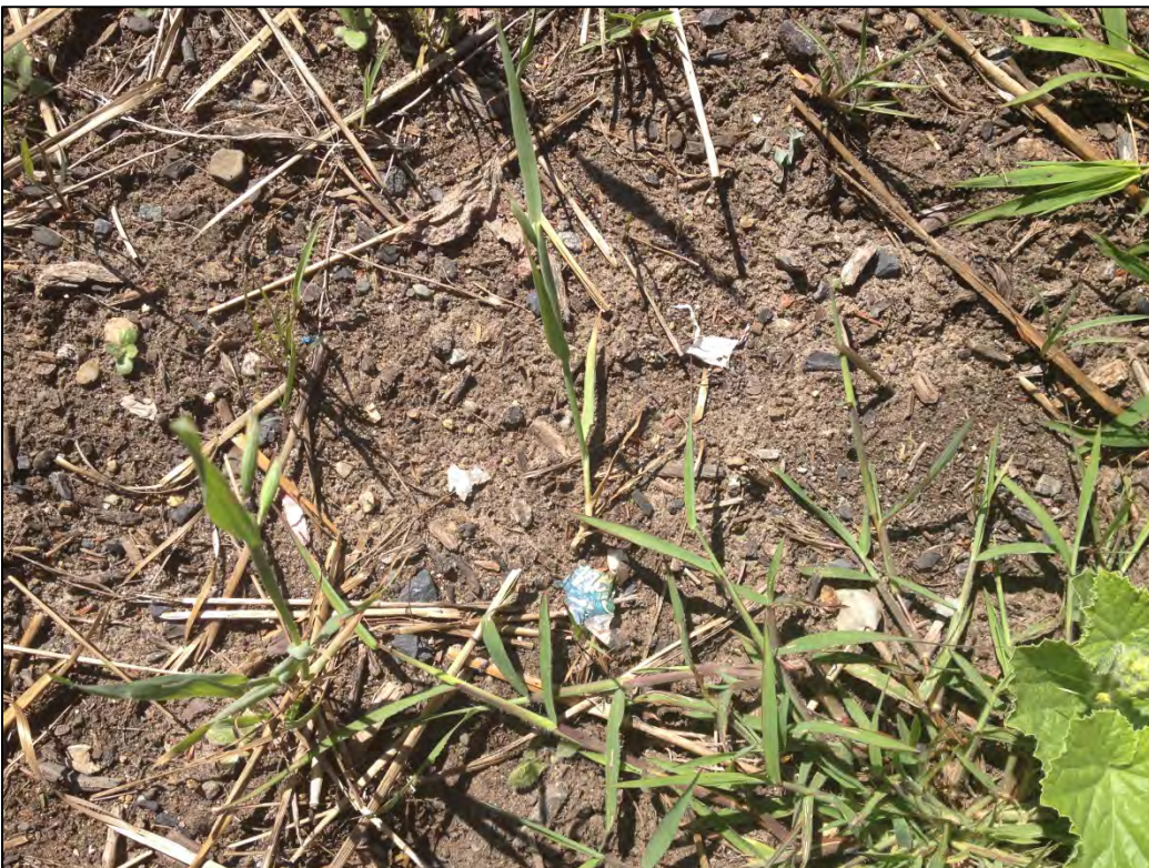
Photo 10: Example of plastic and other debris observed within placed topsoil at several locations within the restored areas along the right of way.
