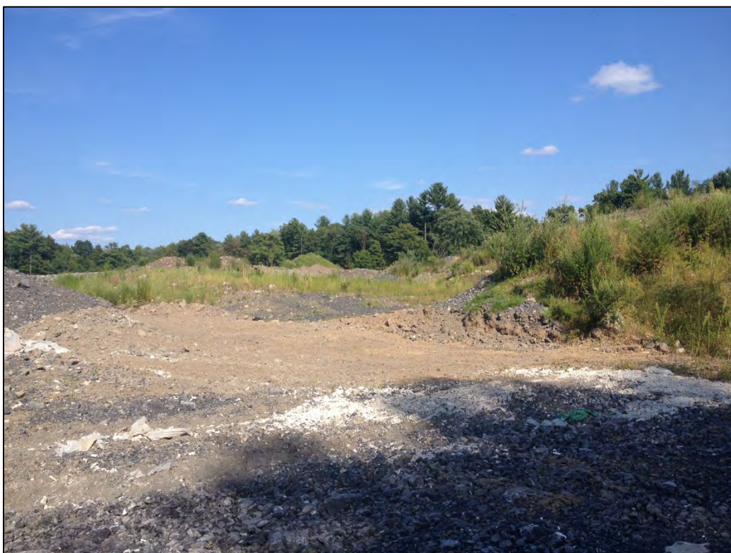
Photo 16: Stone quarry and general equipment washdown area from which stone for the construction access roads was collected.
