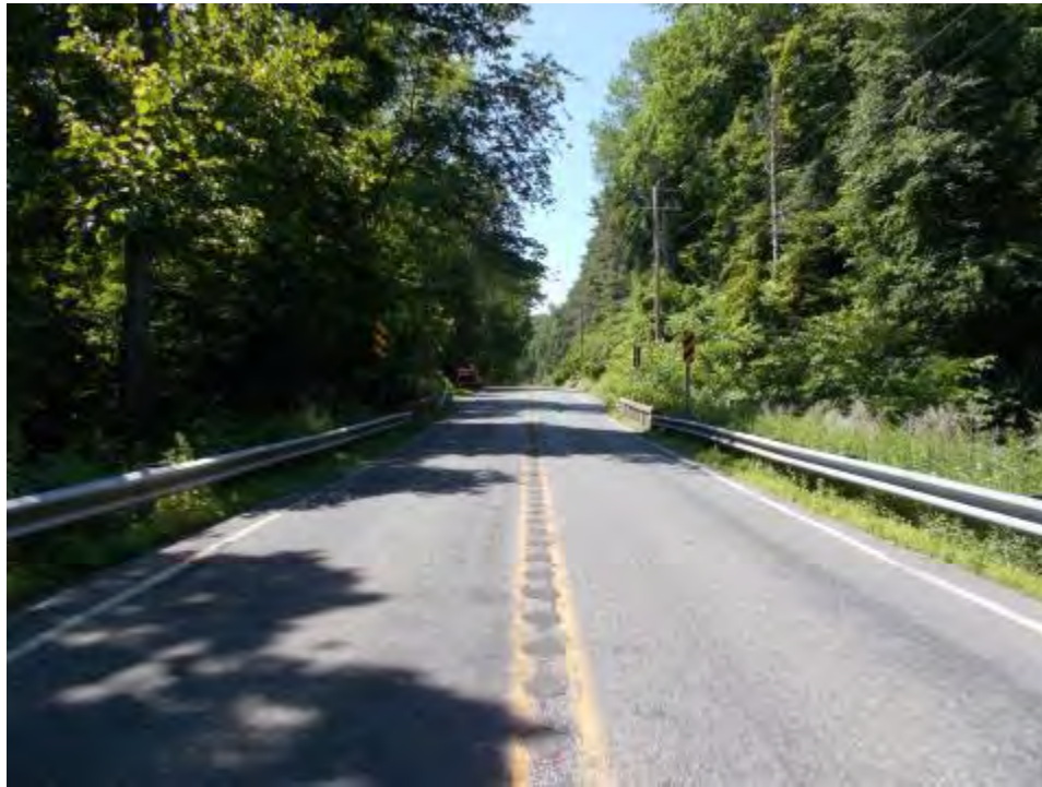
Photograph 1: View of the S.R. 0209 bridge over Adams Creek approach, facing southwest (July 2018).
