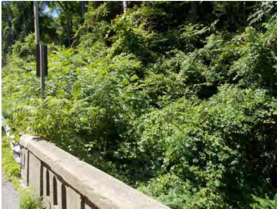
Photograph 7: View of the southwest quadrant of the bridge study area, facing southwest (July 2018).
